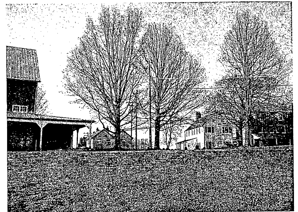
LOOKING NORTH (PARTY BARN TO WEST)
