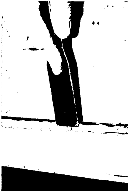
Figure 4d. Reglazing or replacement of the putty requires that the existing putty be removed manually, the glazing points be extracted, the glass removed, and the back putty scraped out. To reglaze, a bed of putty is laid around the perimeter of the rabbet, the pane is pressed into place, glazing points are inserted to hold the pane (shown), and a final seal of putty is beveled around the edge of the glass. Photo: John H. Myers
