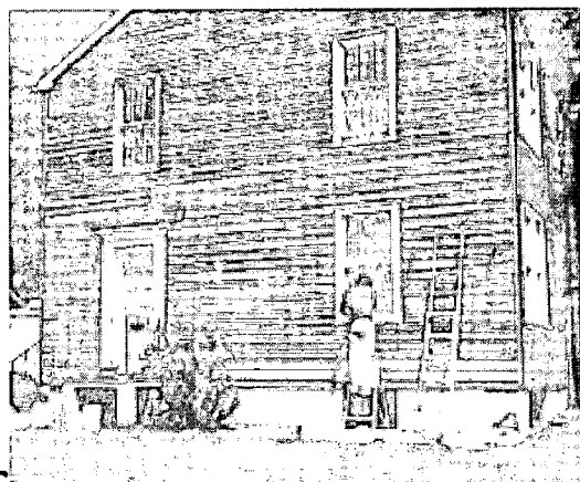
Limited replacement-in-kind of deteriorated wood clapboards.
