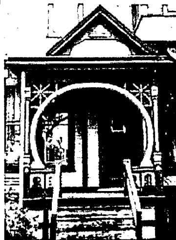
Wood features on porch repaired and preserved during rehabilitation.
