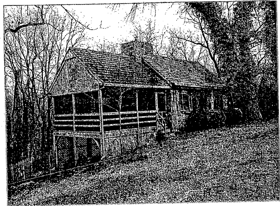
Photo 8 - West and North Elevations
