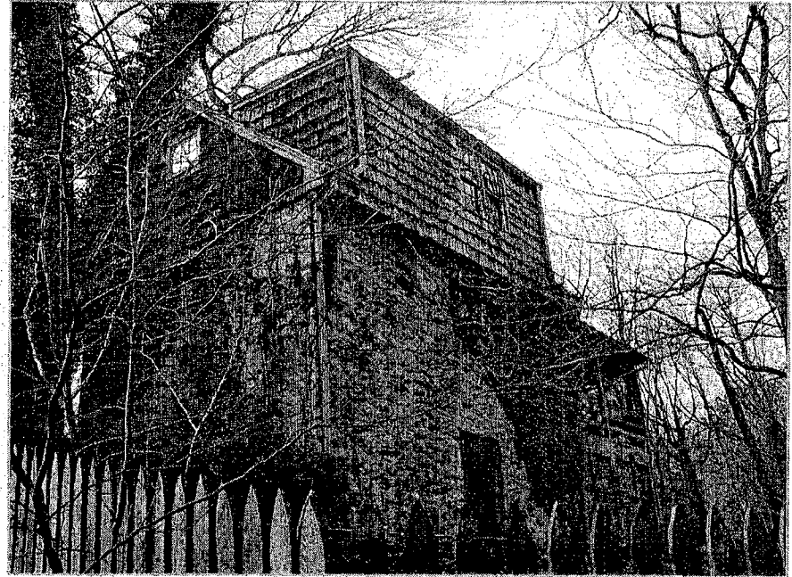
Photo 12 - South and East Elevation
