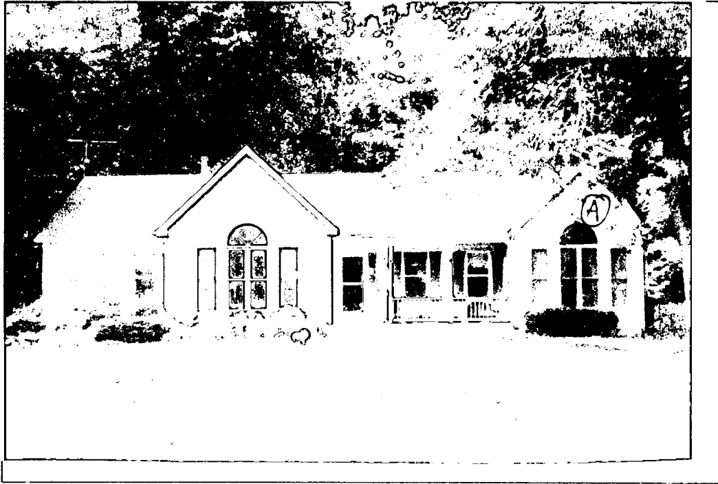
Detail: FRONT VIEW: ADDITION ON THE RIGHT (A) CARPORT ON THE LEFT (B)
