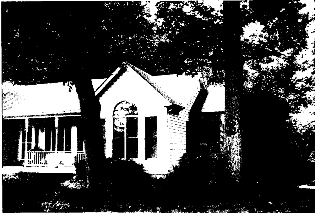
Detail: FRONT RIGHT SIDE VIEW - 2 TREES NEED TO BE REMOVED
