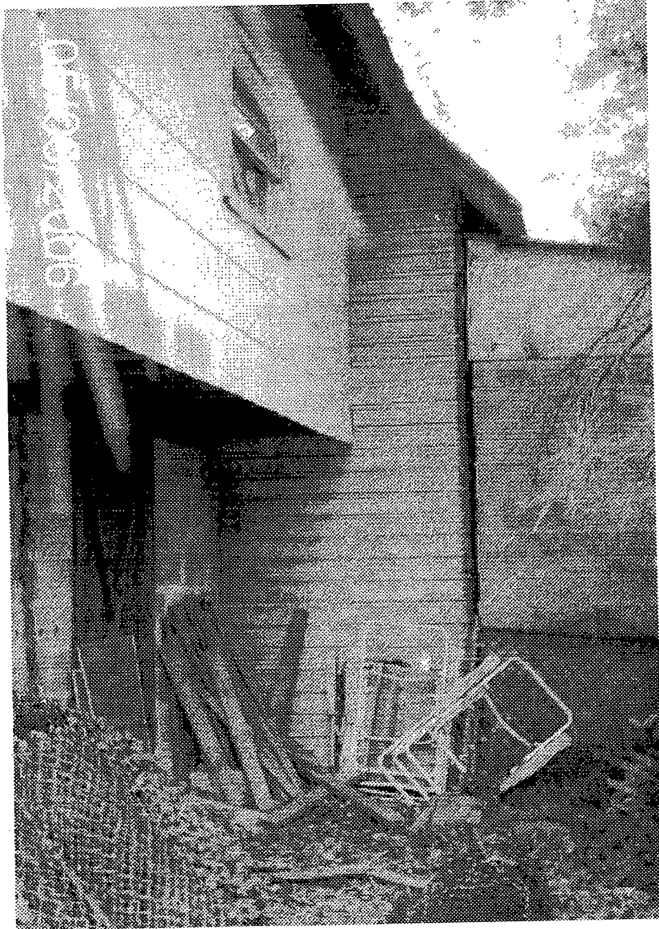
Existing Garage (South Elevation detail)
