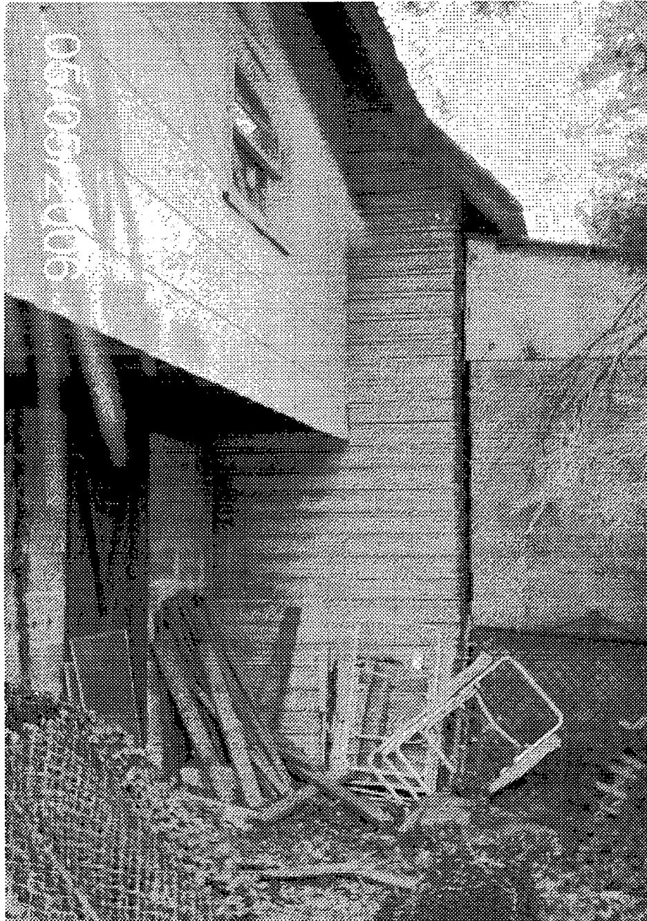
Existing Garage (South Elevation detail)
