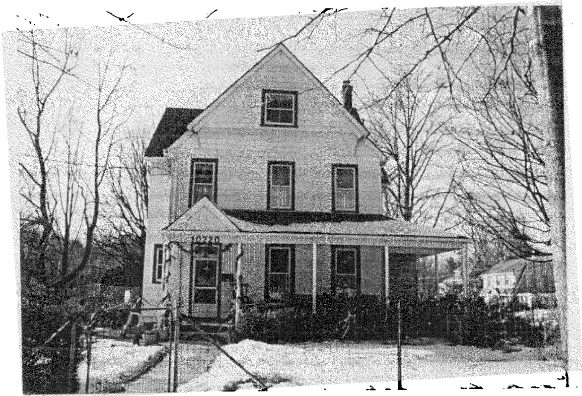
Eastern elevation today
