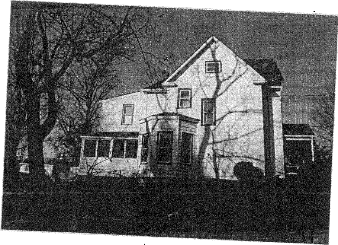
South elevation today
