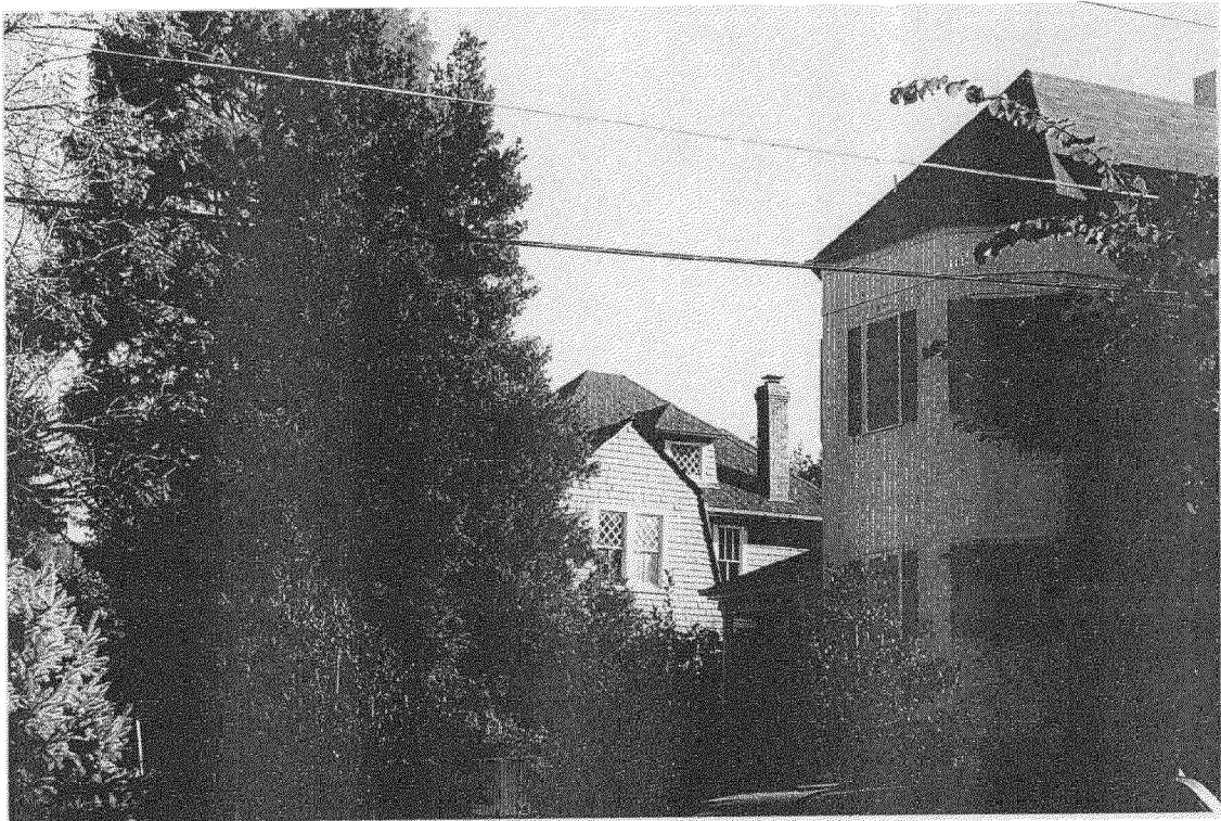
South side (viewed from Baltimore Ave.)
