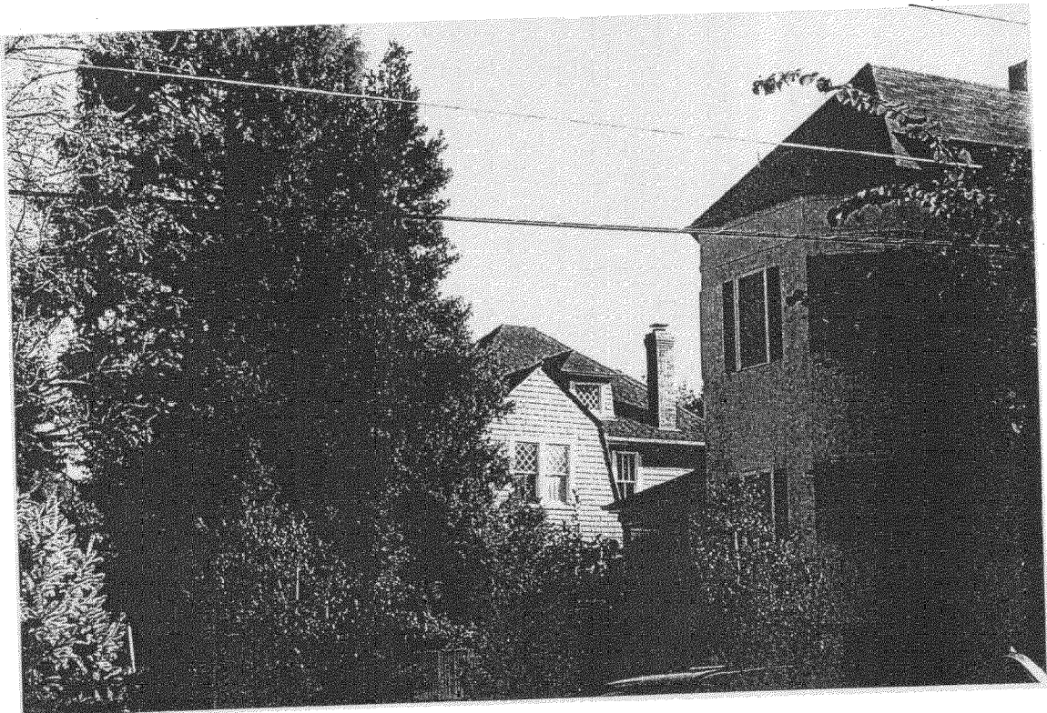
South side (viewed from Baltimore Ave.)
