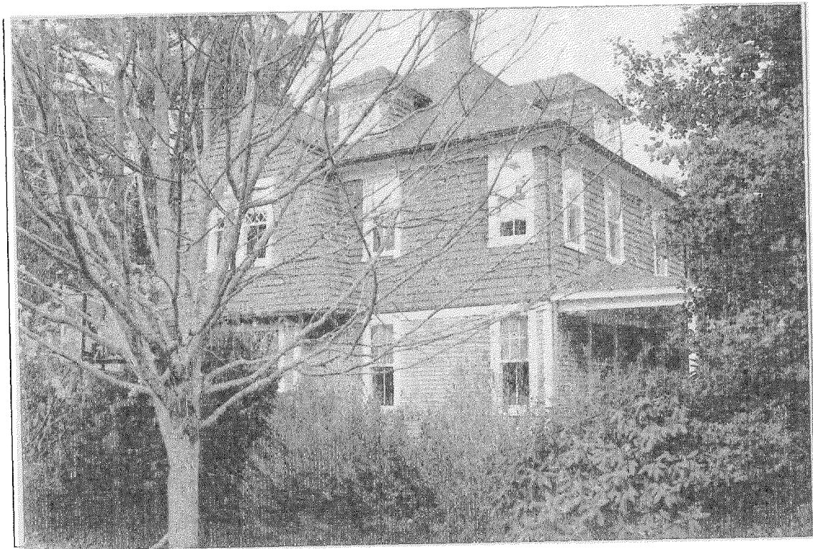
Detail: side of house (south)
