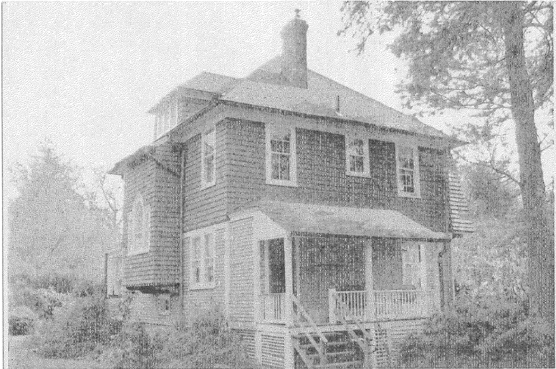
Detail: back of house (west) - porch and pantry to be removed
