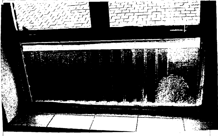
Detail: Example of window condition
