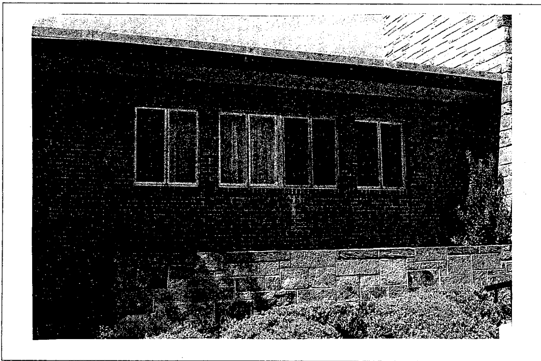
Detail: Parlor exterior 4 windows aluminum frame
