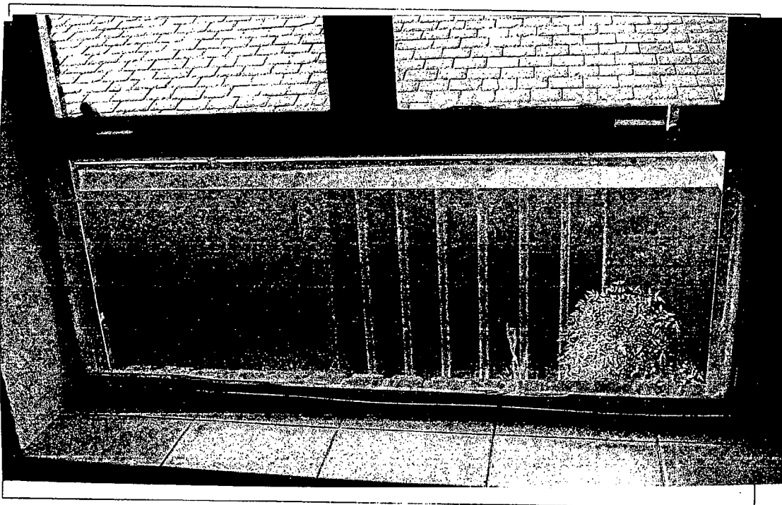
Detail: Example of window condition
