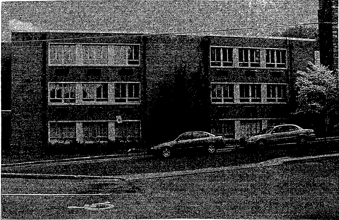
Detail: View from Mitchell St Southside
