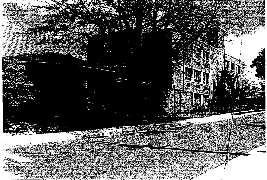
Detail: view from Army + Mitchell St SW corner
