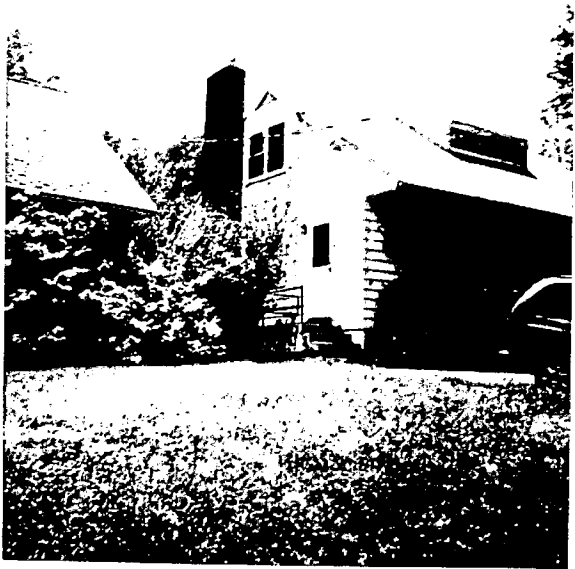
LEFT SIDE OF HOUSE FROM FRONT YARD.
