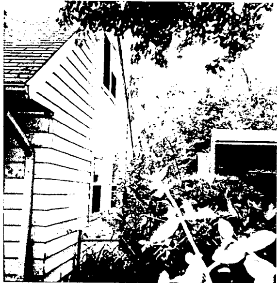
RIGHT SIDE OF HOUSE FROM FRONT YARD.
