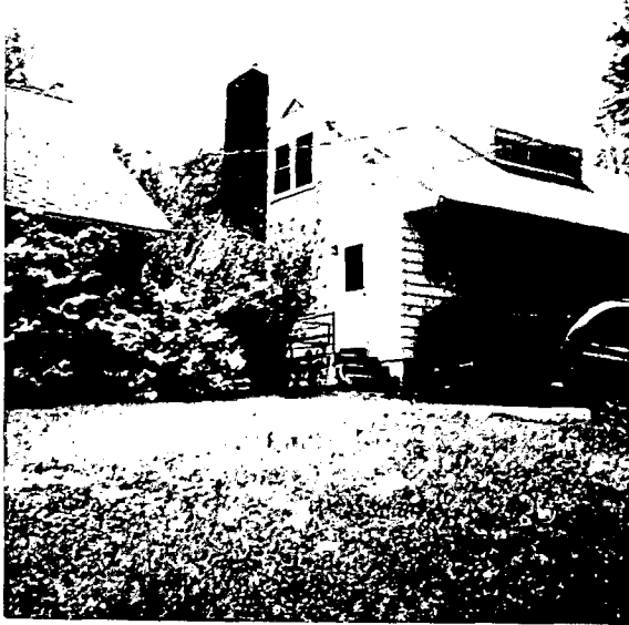
LEFT SIDE OF HOUSE FROM FRONT YARD.
