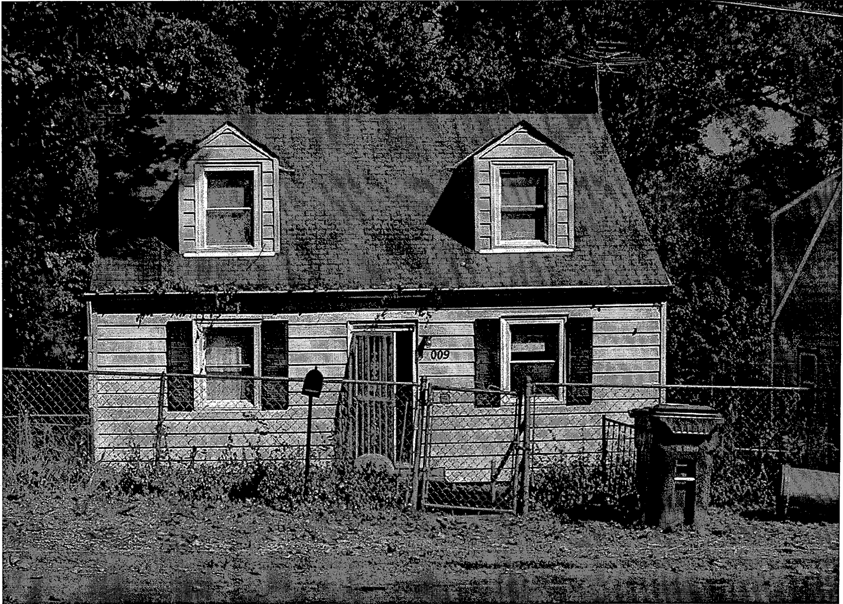
FRONT ELEVATION TAKEN FROM MENLO AVENUE. EXISTING RESIDENCE FROM TOP OF CMU BASEMENT WALL TO BE REMOVED
