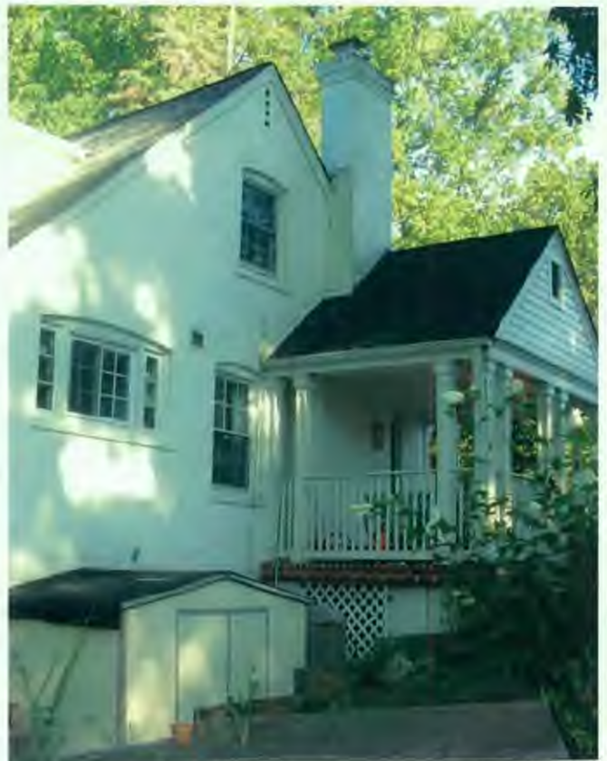
REAR OF EXISTING PORCH
