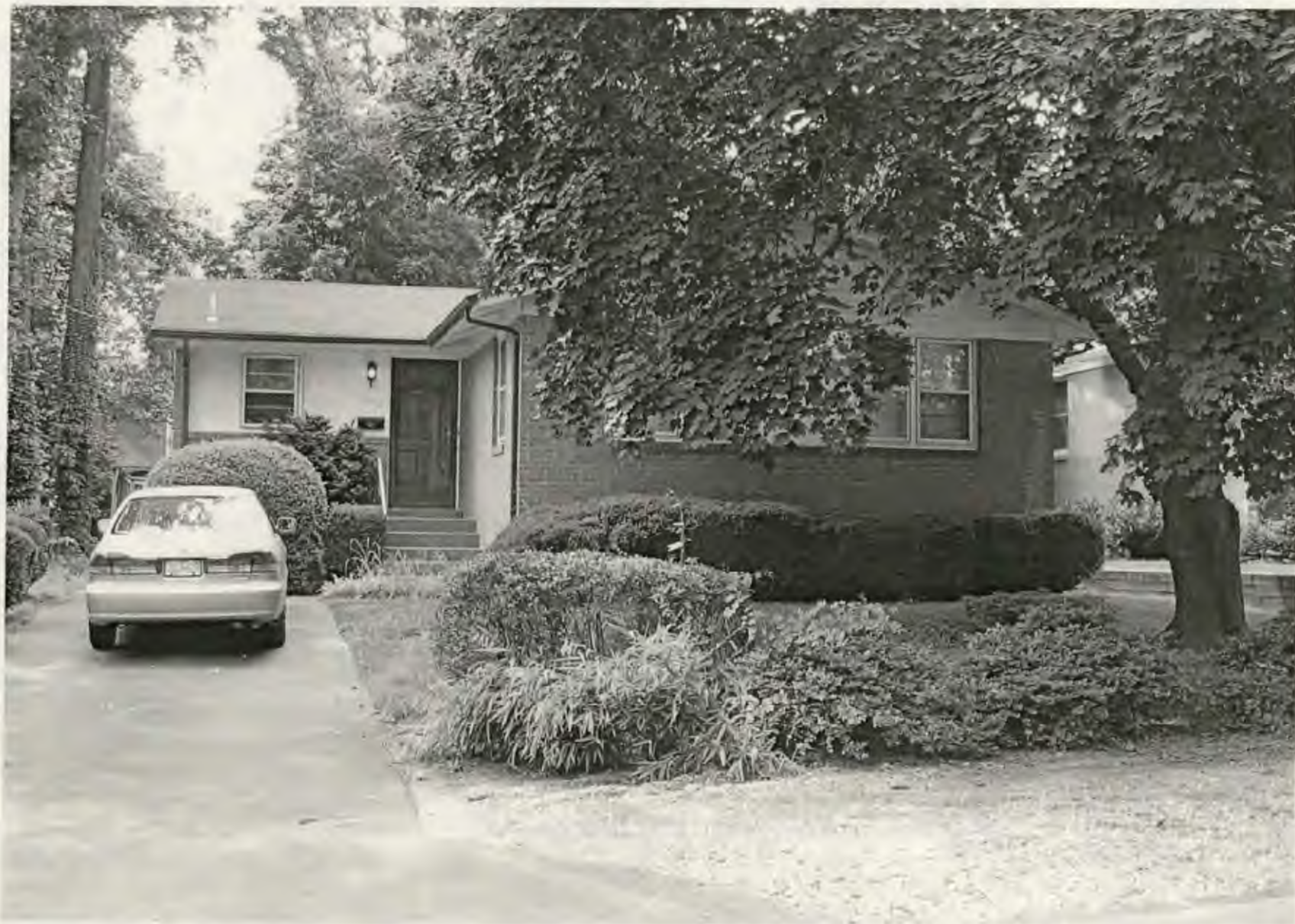
10102 Grant Avenue View of Property Fronting BenAvram Residence
