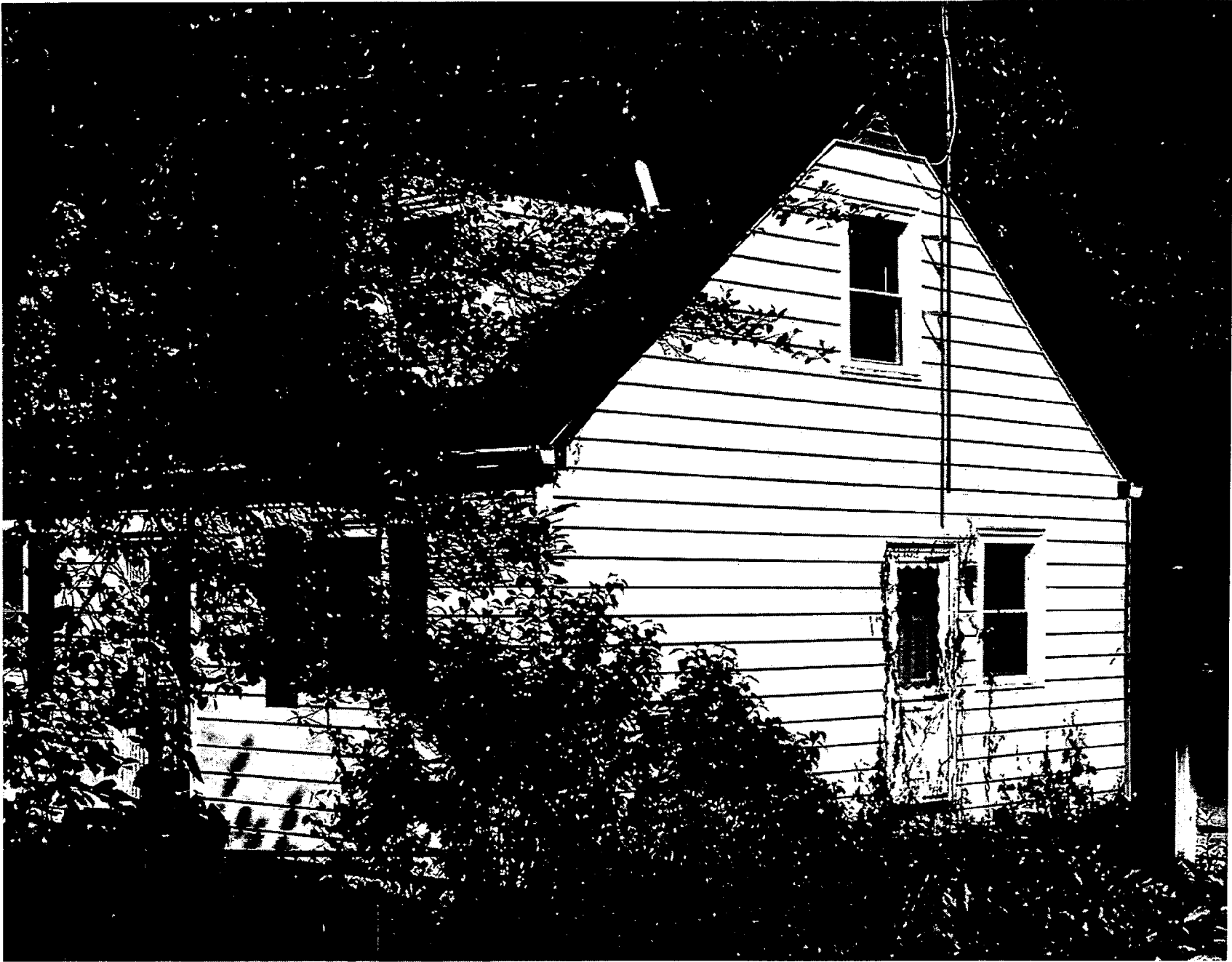
RIGHT ELEVATION TAKEN FROM MENLO AVENUE. EXISTING RESIDENCE FROM TOP OF CMU BASEMENT WALL TO BE REMOVED
