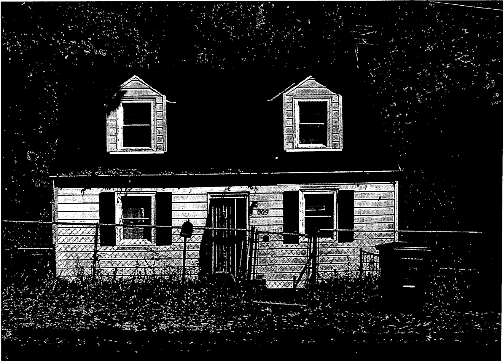
FRONT ELEVATION TAKEN FROM MENLO AVENUE. EXISTING RESIDENCE FROM TOP OF CMU BASEMENT WALL TO BE REMOVED
