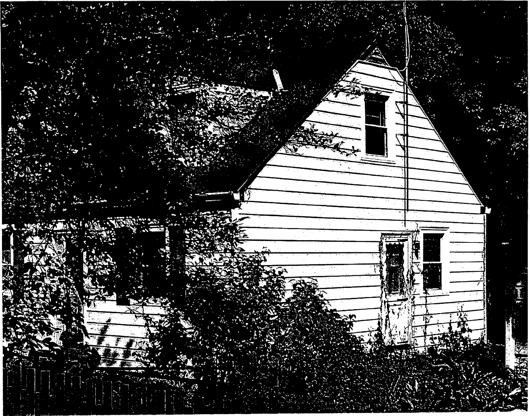
RIGHT ELEVATION TAKEN FROM MENLO AVENUE. EXISTING RESIDENCE FROM TOP OF CMU BASEMENT WALL TO BE REMOVED
