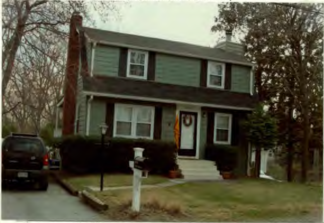
Detail: 10113 Grant Replacement Siding
