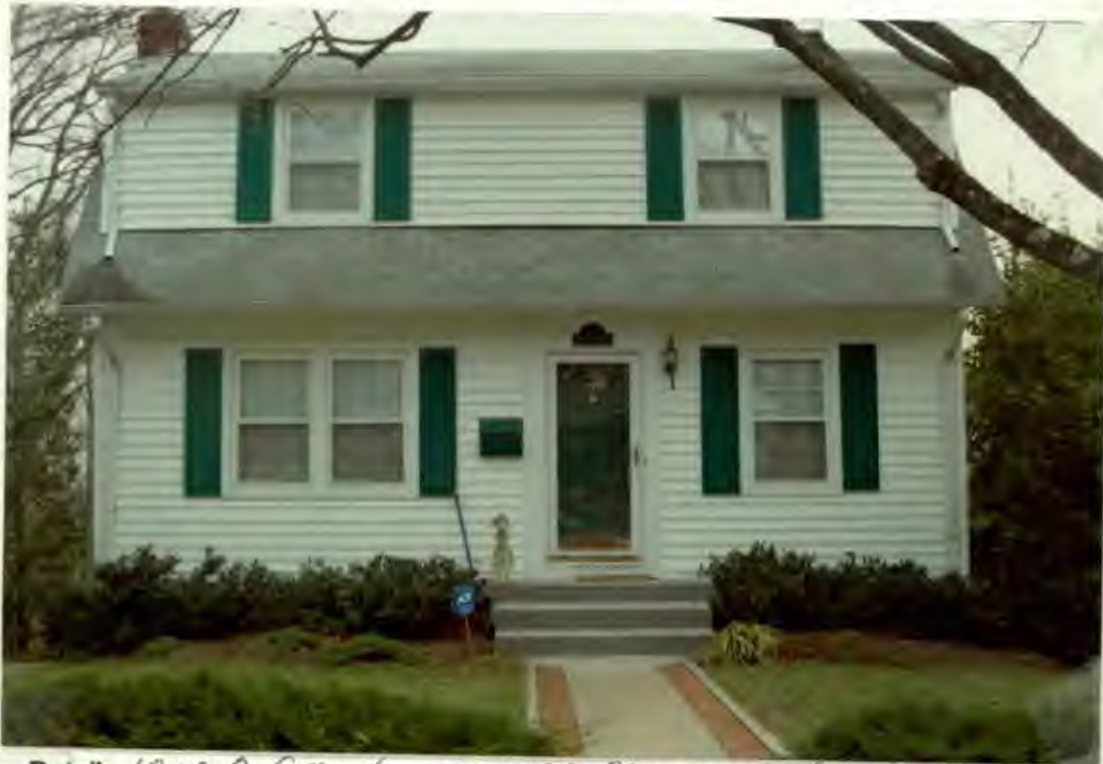
Detail: 10109 Grant Replacement Siding
