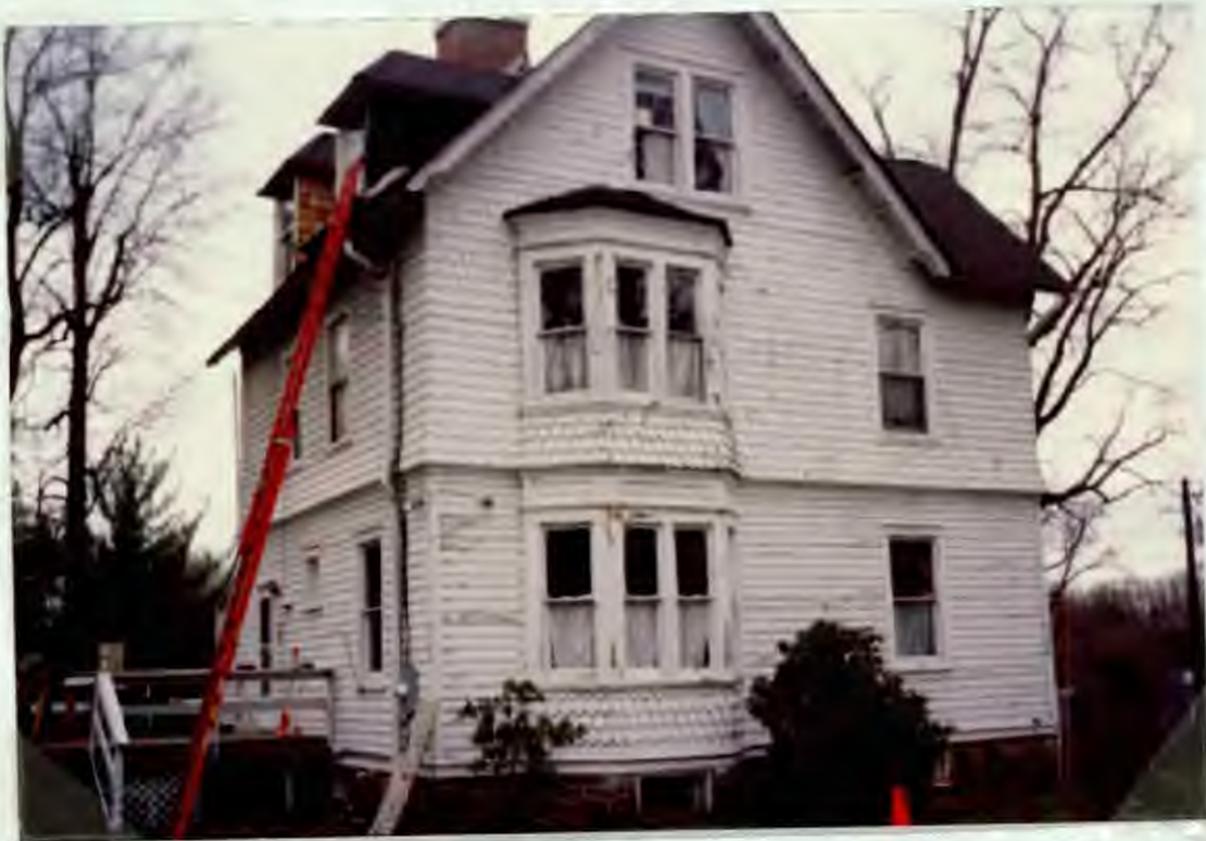
3120 Lee Street pre-paint job View from Lee Street
