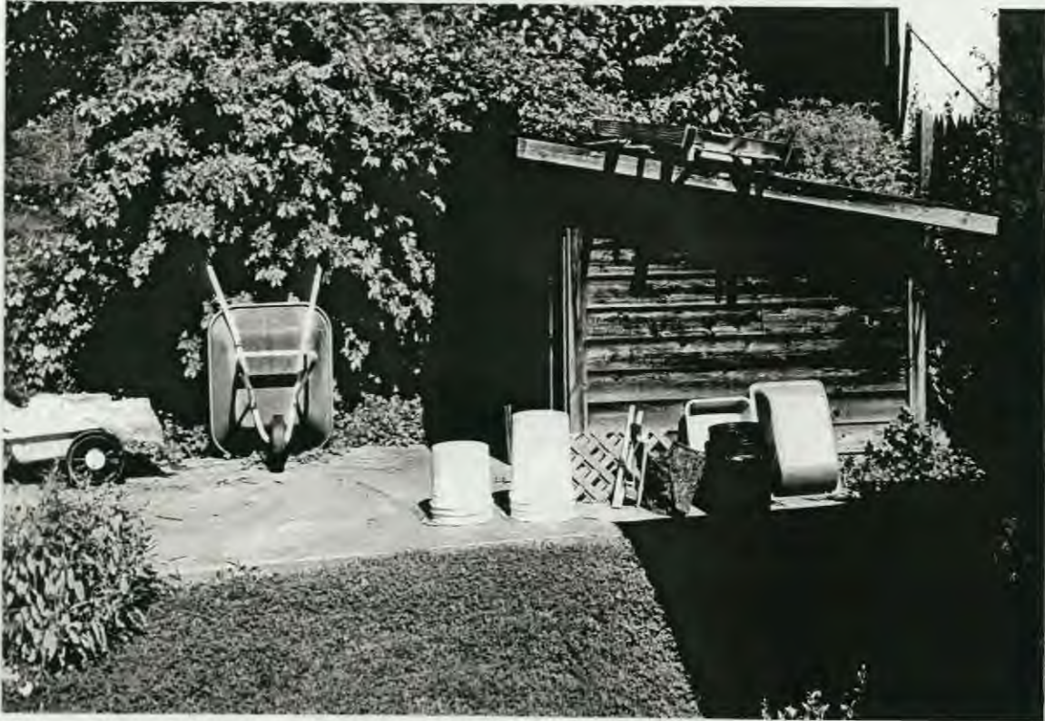
Existing Shed and Concrete Slab East Side
