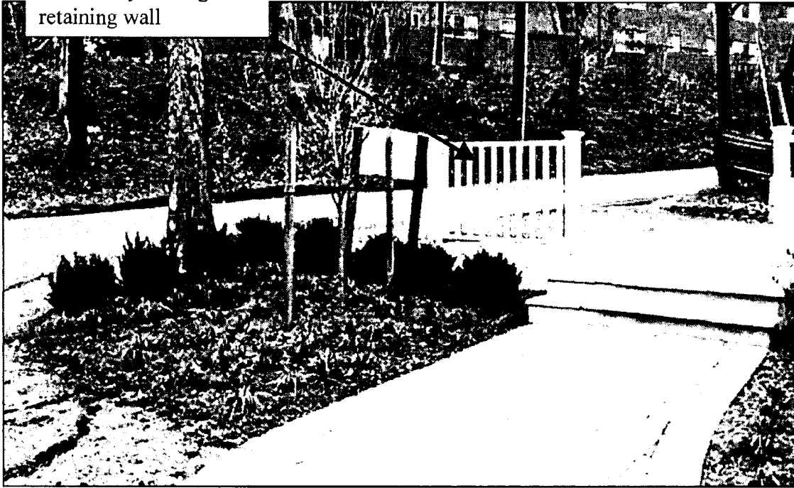
Install wood fence on retaining wall along side property line (3-4' at front yard, 6' max at rear)
