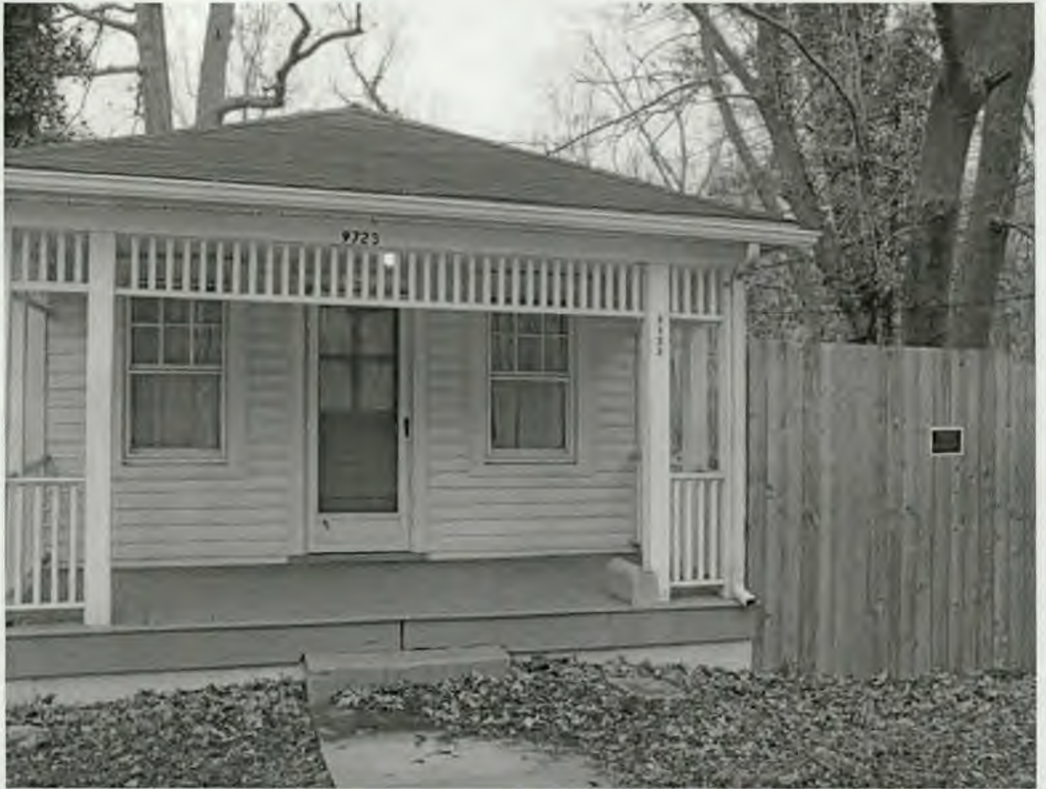
front door that was removed
