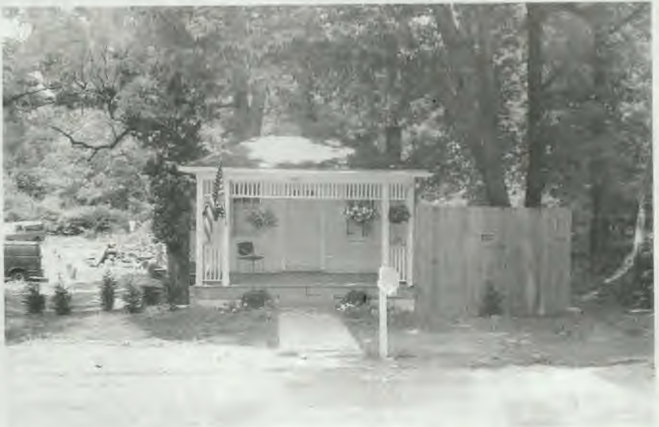
replacement front door
