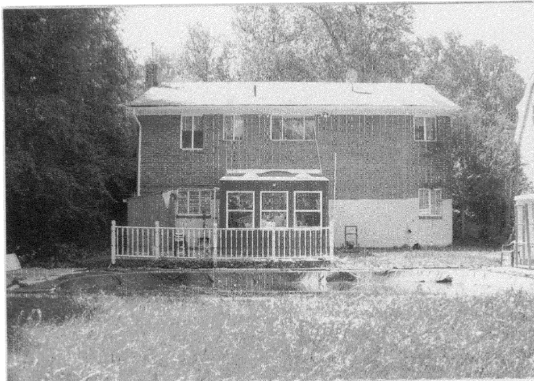
Detail: Rear of house
