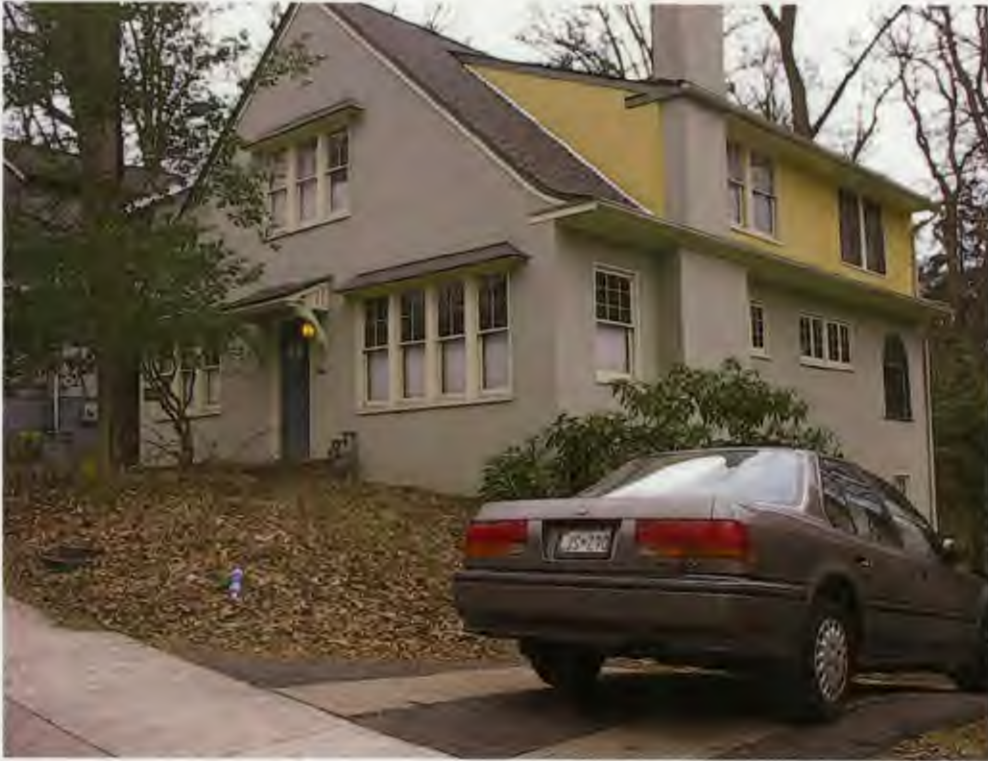
Existing right façade of 7330 Piney Branch Road, Takoma Park, MD 20912
