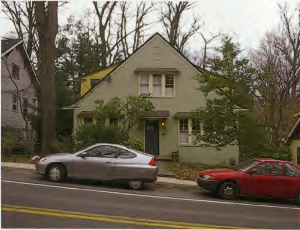
Existing front façade of 7300 Piney Branch Road, Takoma Park, MD 20912
