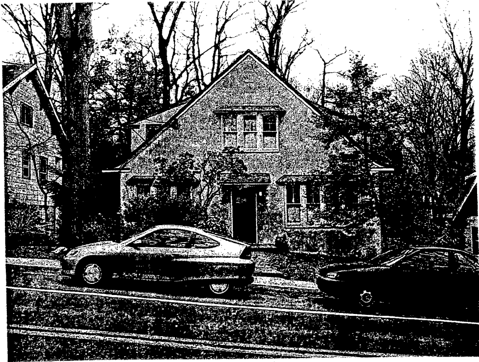
Existing front façade of 7300 Piney Branch Road, Takoma Park, MD 20912
