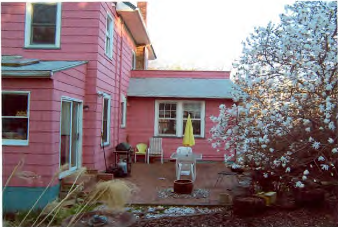
SOUTHWEST CORNER OF BUILDING
