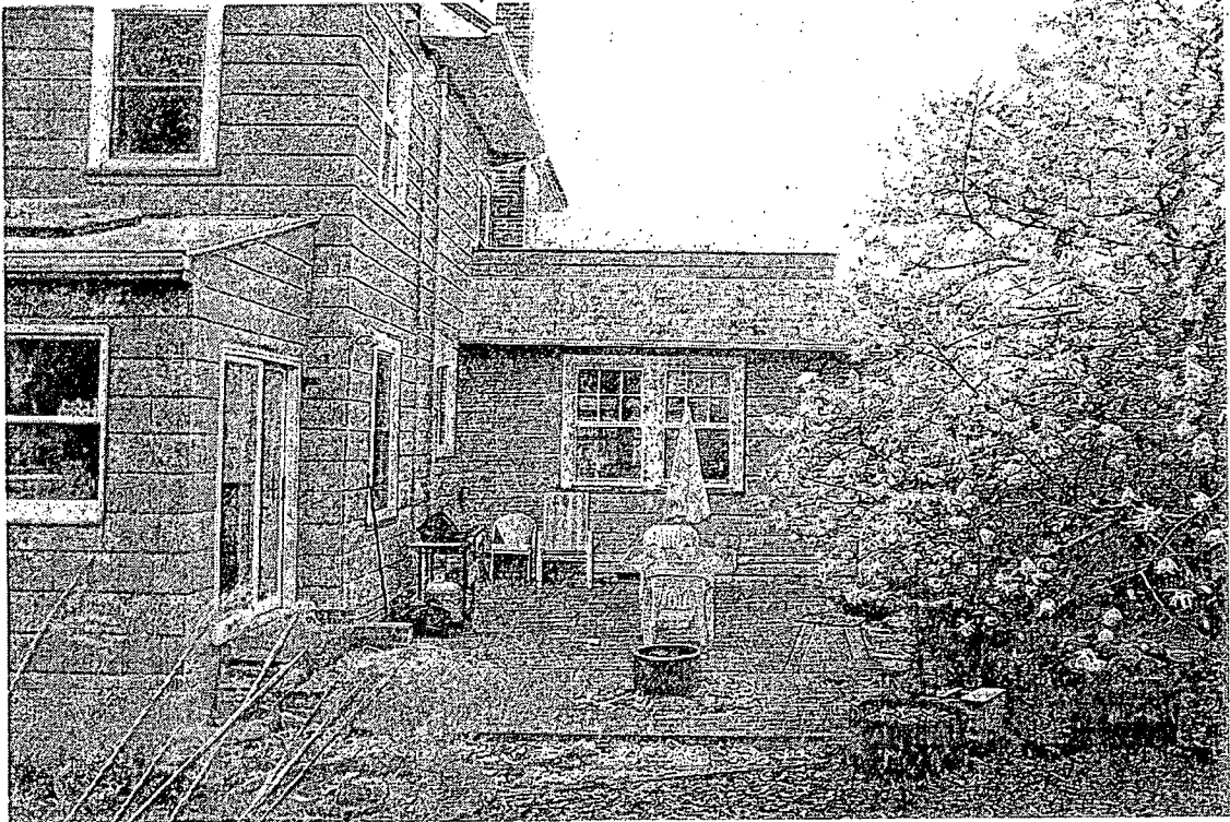
SOUTHWEST CORNER OF BUILDING
