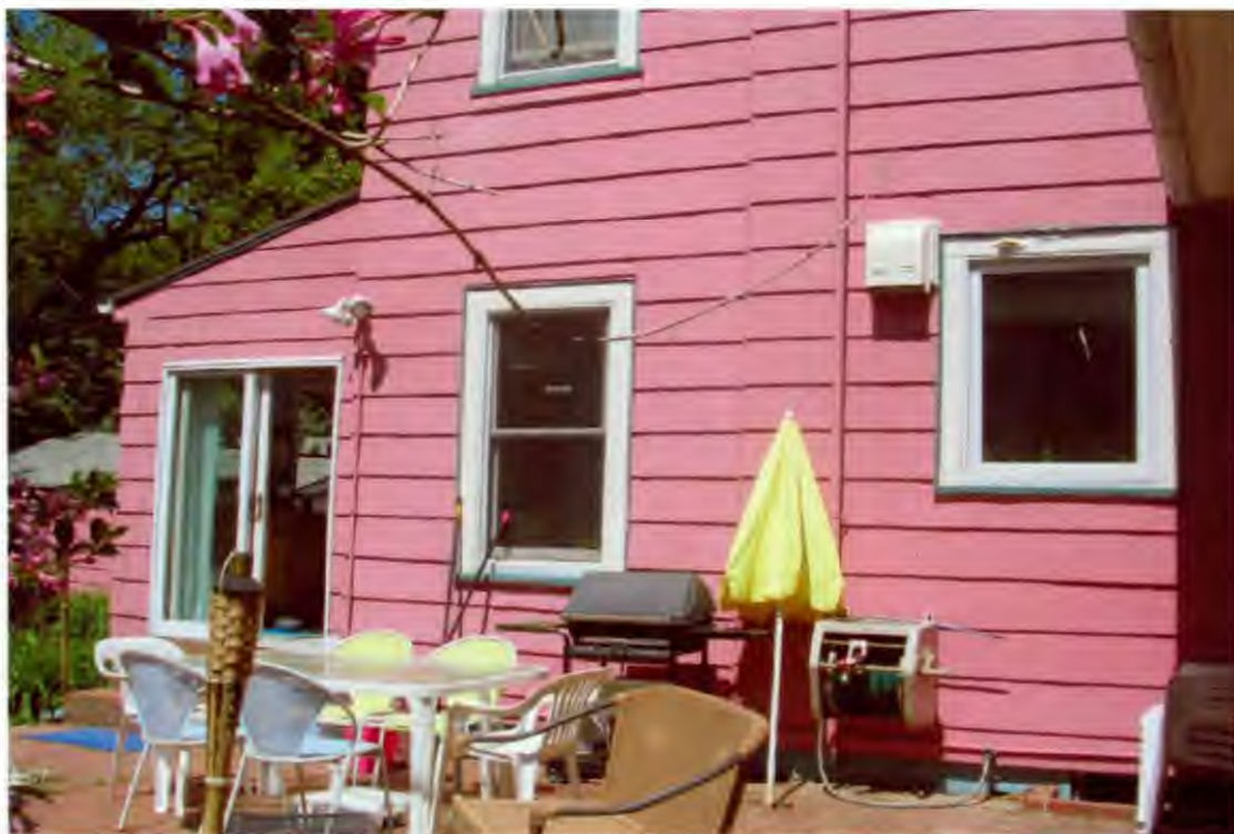
SOUTH SIDE OF BUILDING
