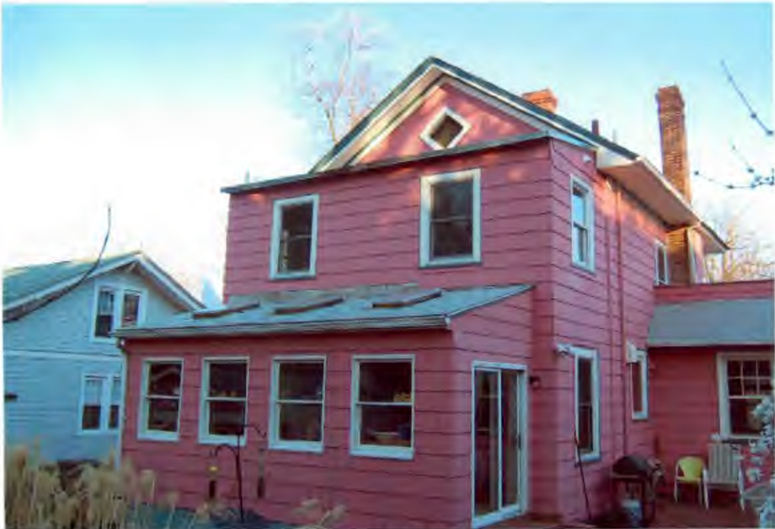
WEST SIDE OF BUILDING
