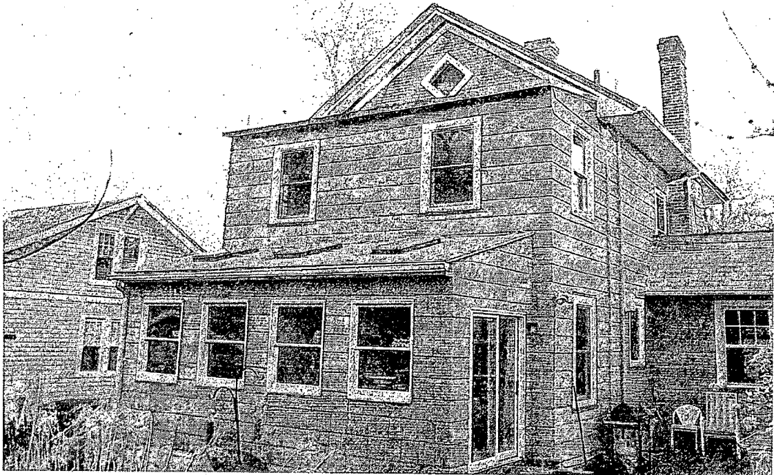
WEST SIDE OF BUILDING
