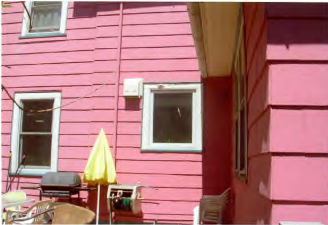
SOUTHSIDE DETAILS OF BUILDING
