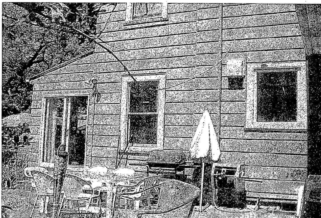
SOUTH SIDE OF BUILDING
