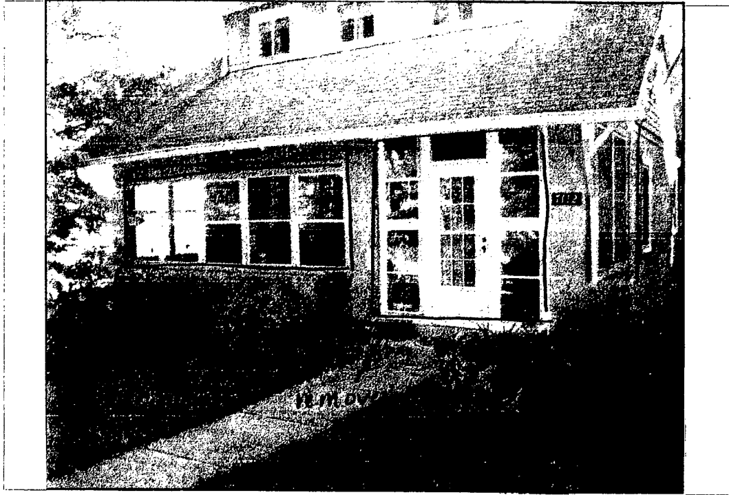
Detail: Front Facade - North
