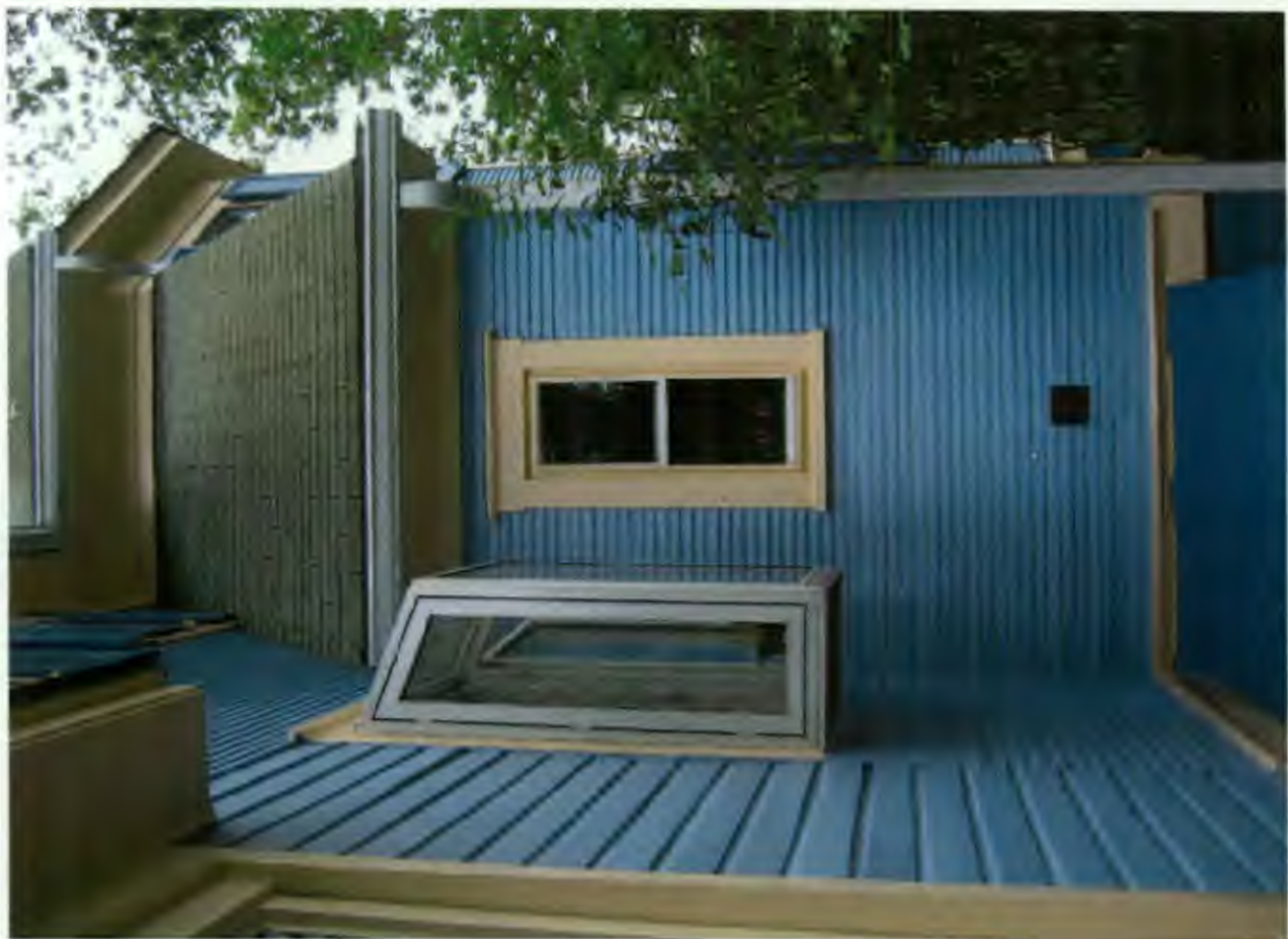
DETAIL OF 1987 RENOVATION
