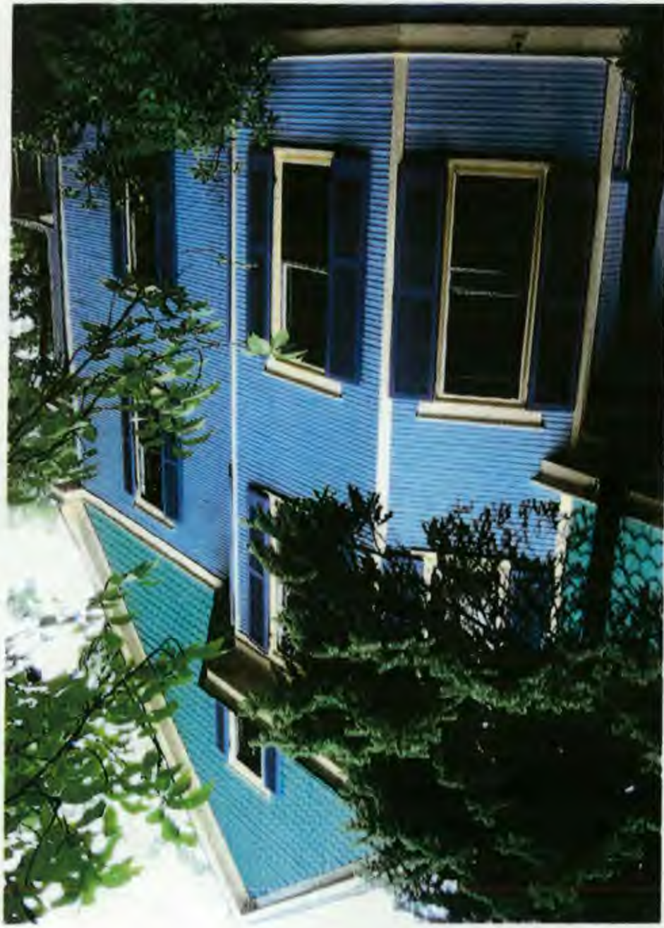
VIEW OF NORTHEAST SIDE FACADE
