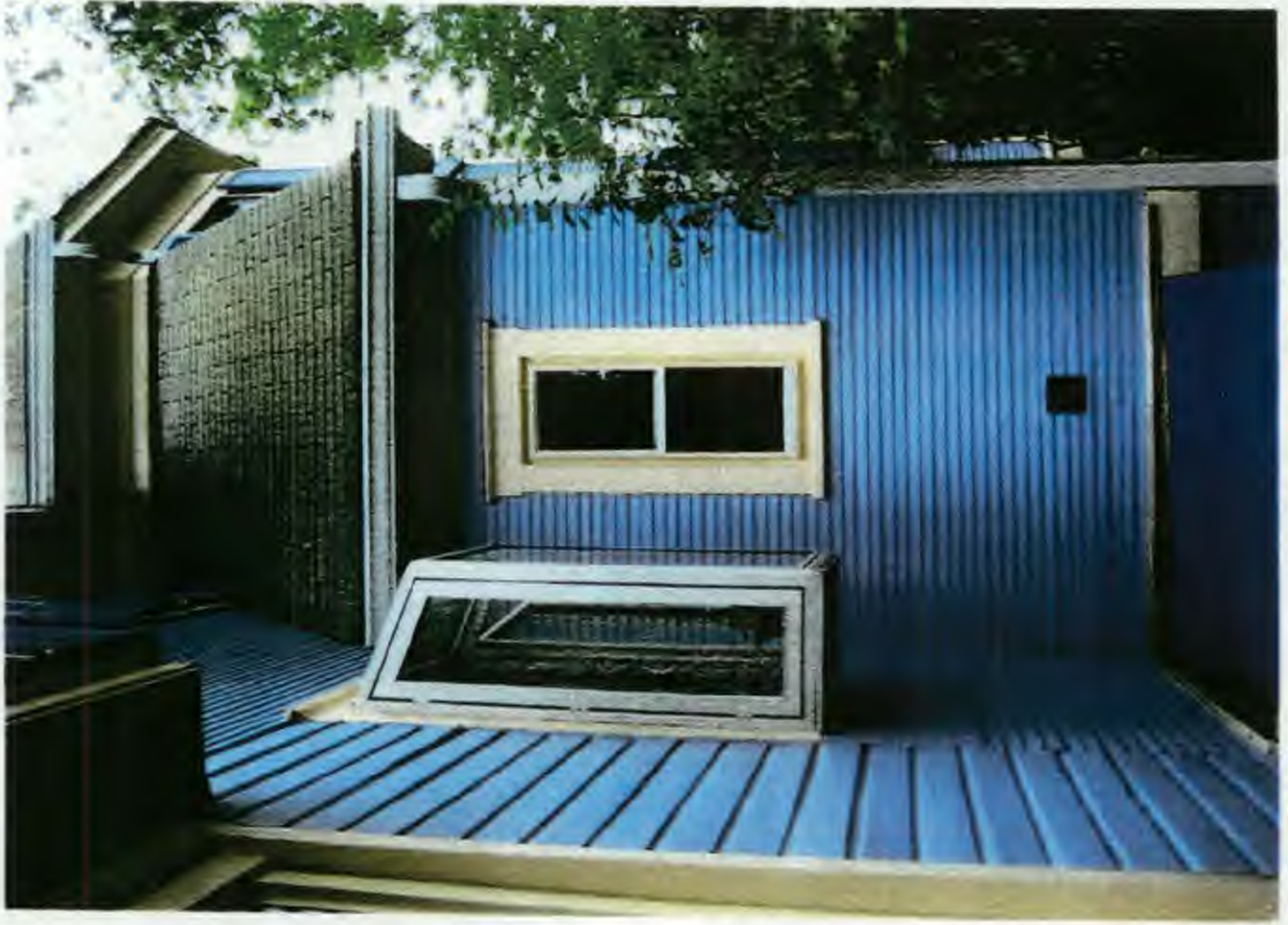
DETAIL OF 1982 RENOVATION
