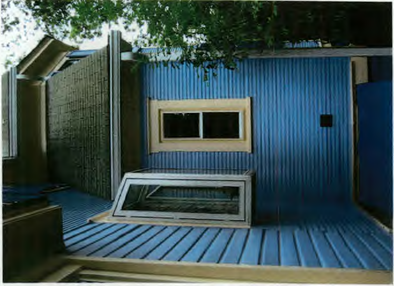
DETAIL OF 1983 RENOVATION
