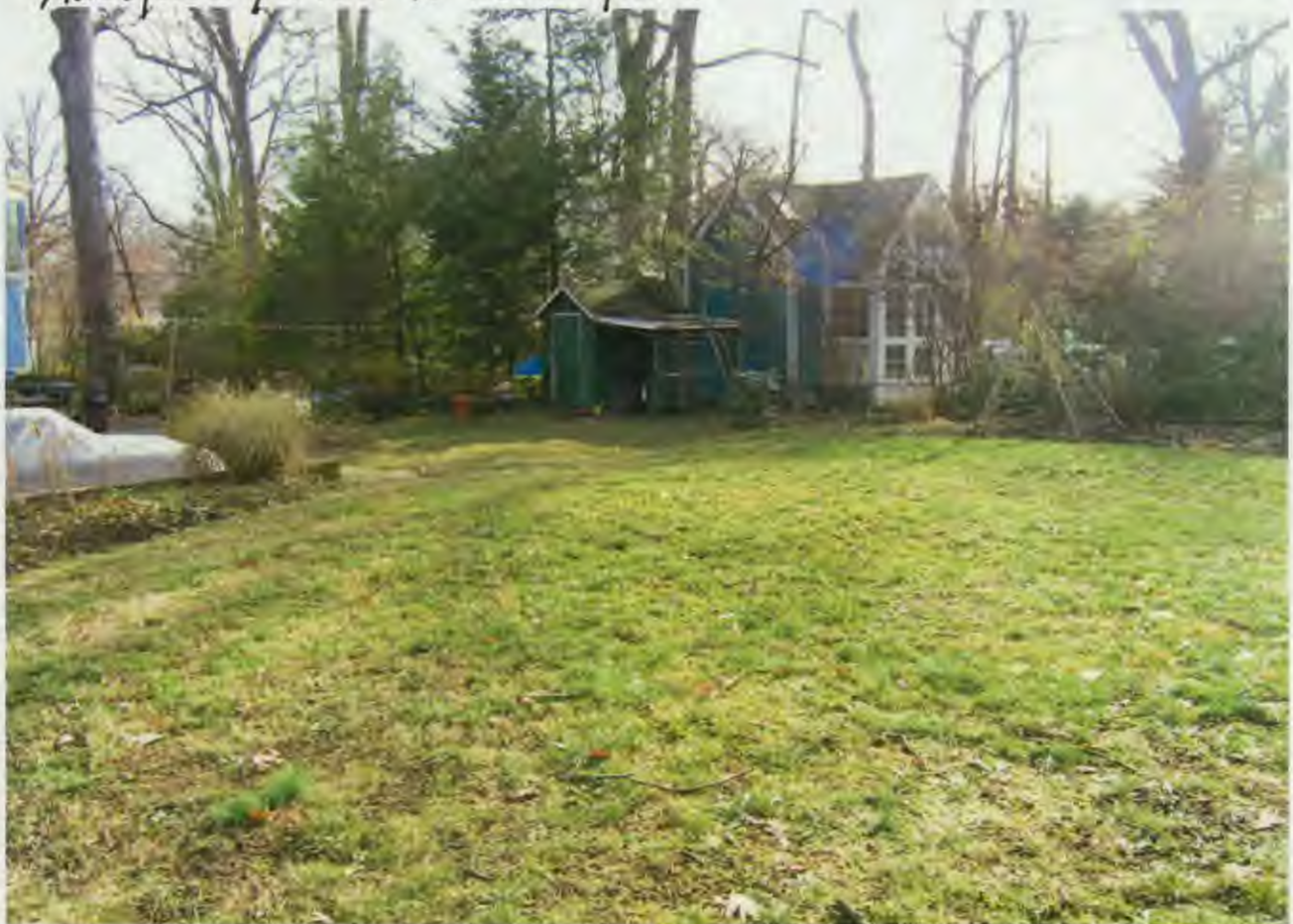
ex. rear yard and shed (to be demolished)
