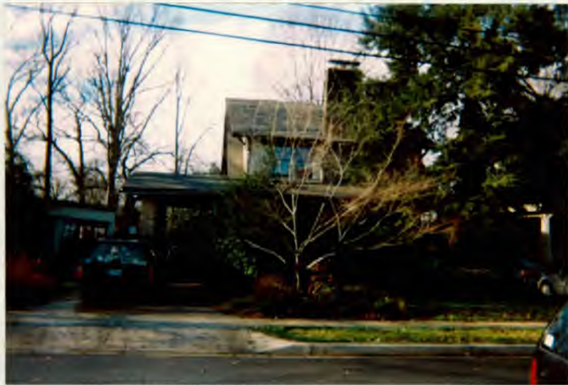
② N/NE FRONT FACADE OF HOUSE AND TWO-CAR GARAGE
