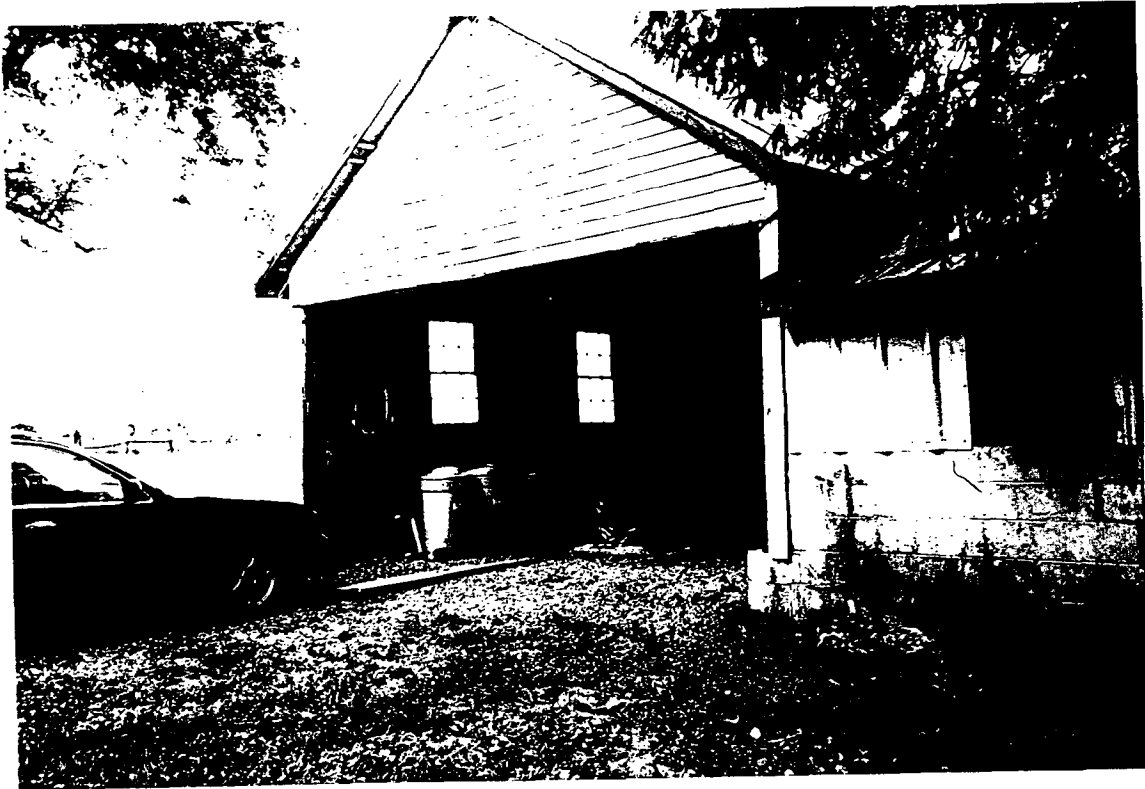
Photo A-1 Front view of garage w/o door
