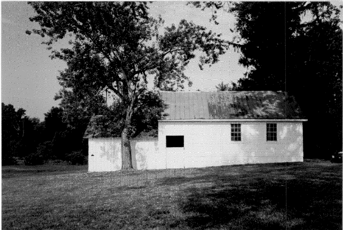
Photo E - side view of garage (painted)
