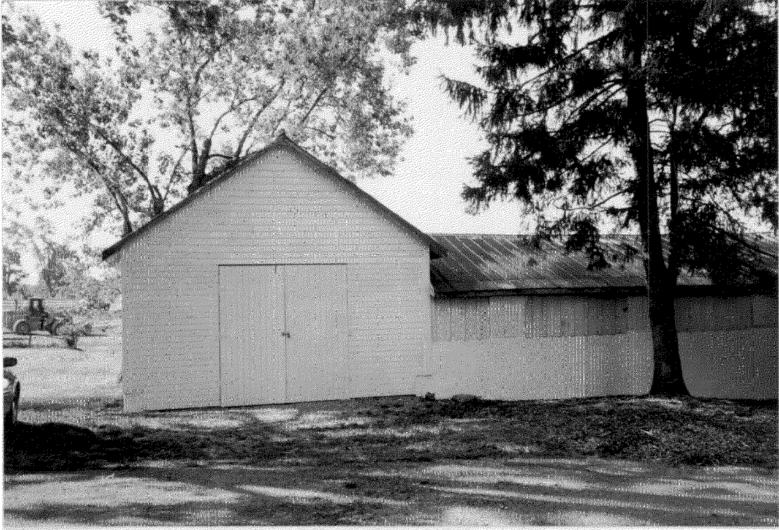
Photo D - view of new front garage doors
