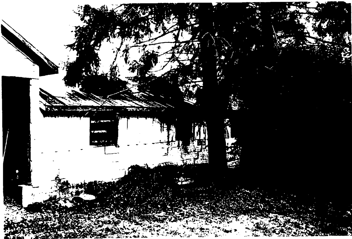
Photo A-2 view of front aluminum siding
