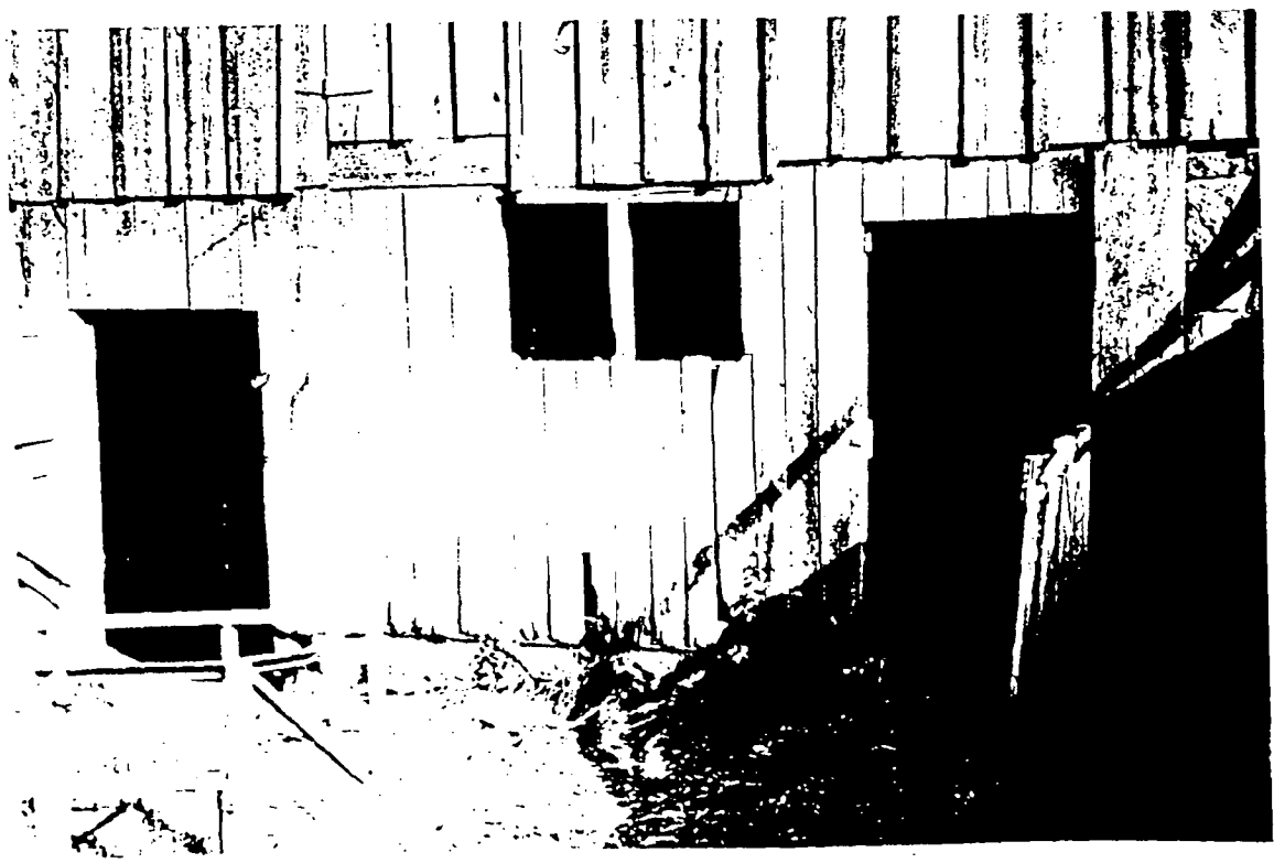
Photo 4 - Detail of area to be restored
