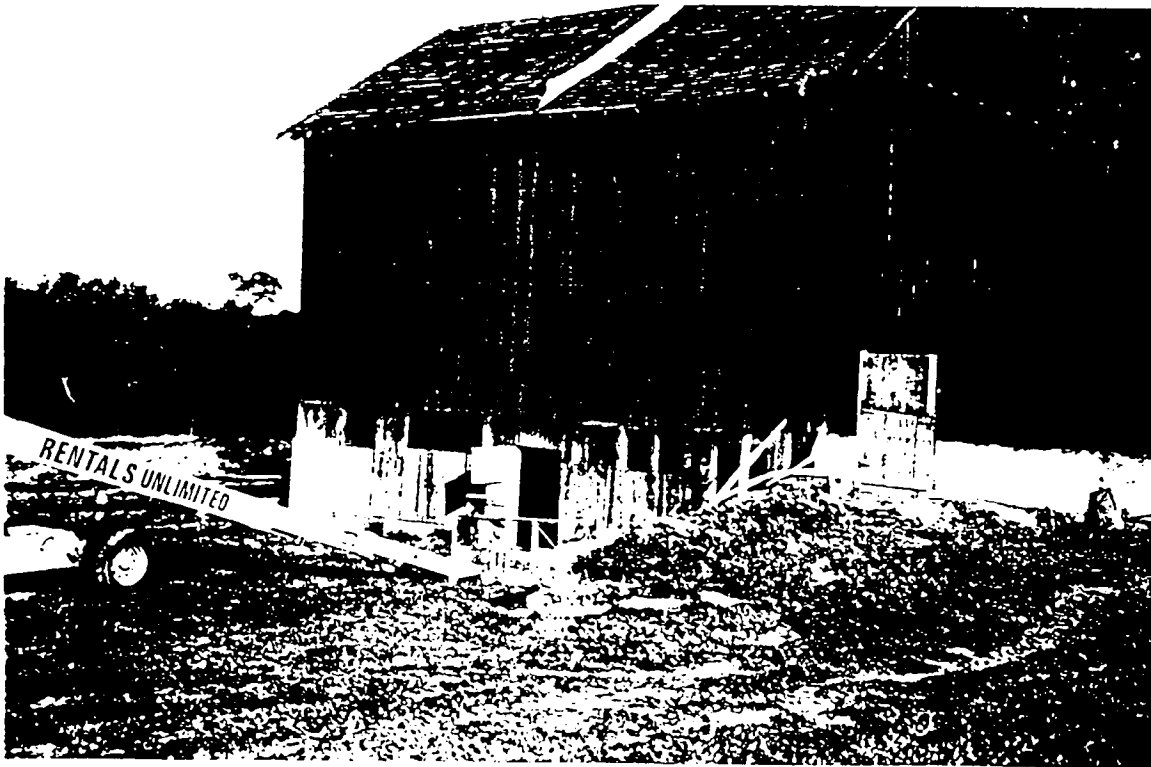
Photo 2 - Barn nearly completed & painted south side of barn
