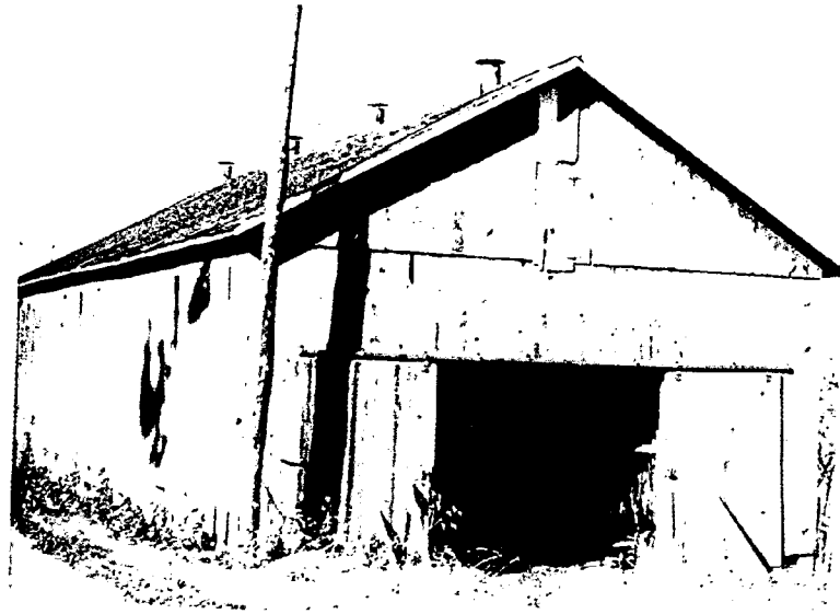
Fig. 8.10 An Air-Cured Tobacco barn typical of south-central Wisconsin. Note the metal ventilators along the ridge.
