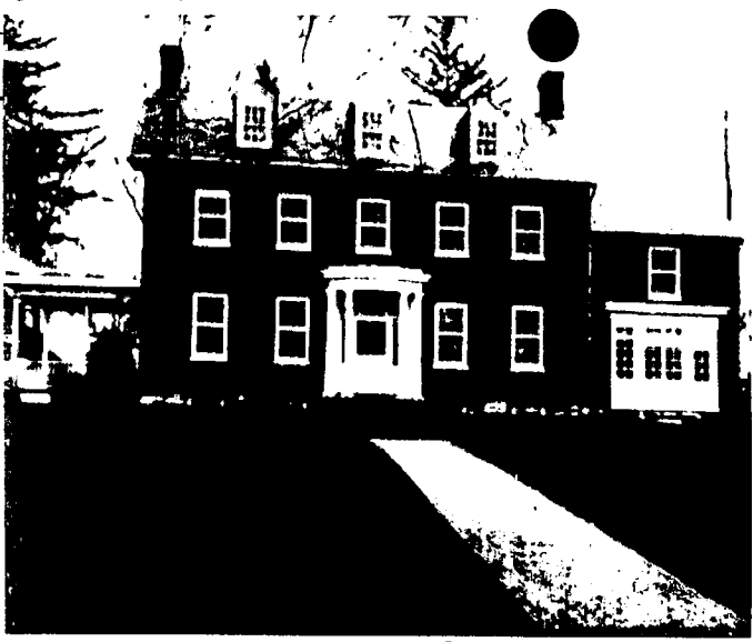
Front view of Manor House
