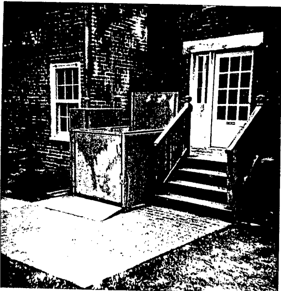
Rear showing existing porch and chair lift
