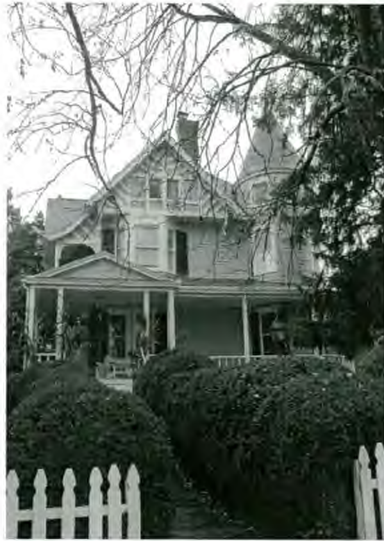
Front elevation of 10400 Montgomery Avenue
