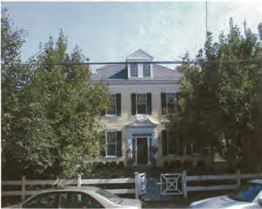
Photo 1: WEST SIDE @ MONTGOMERY AVENUE
