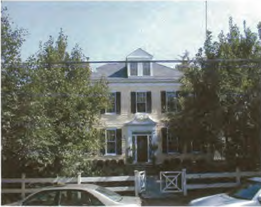
Photo 1: WEST SIDE @ MONTGOMERY AVENUE
