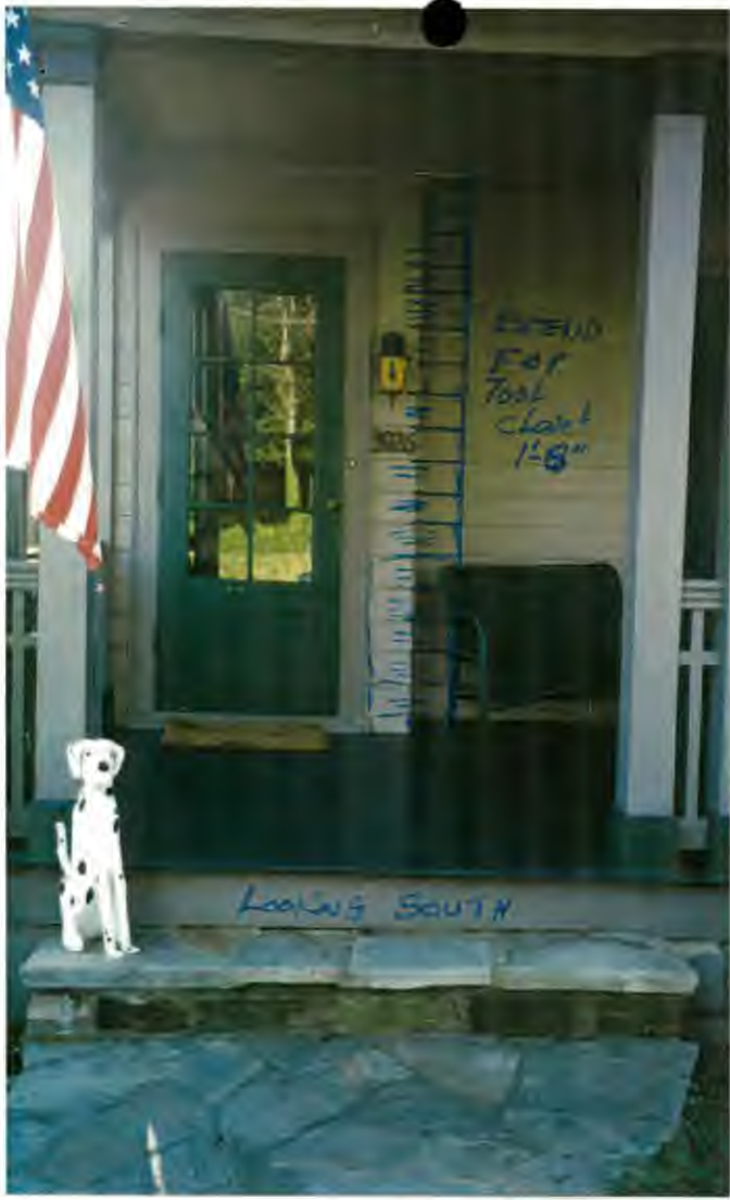
Looking South Tool Closet to the West of Front Porch
