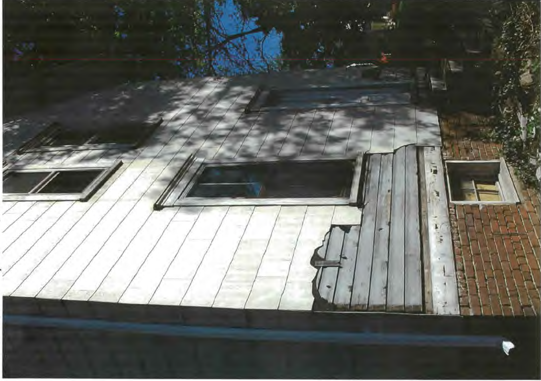
EXISTING HOUSE, LOT 5B, VIEW OF FRONT
