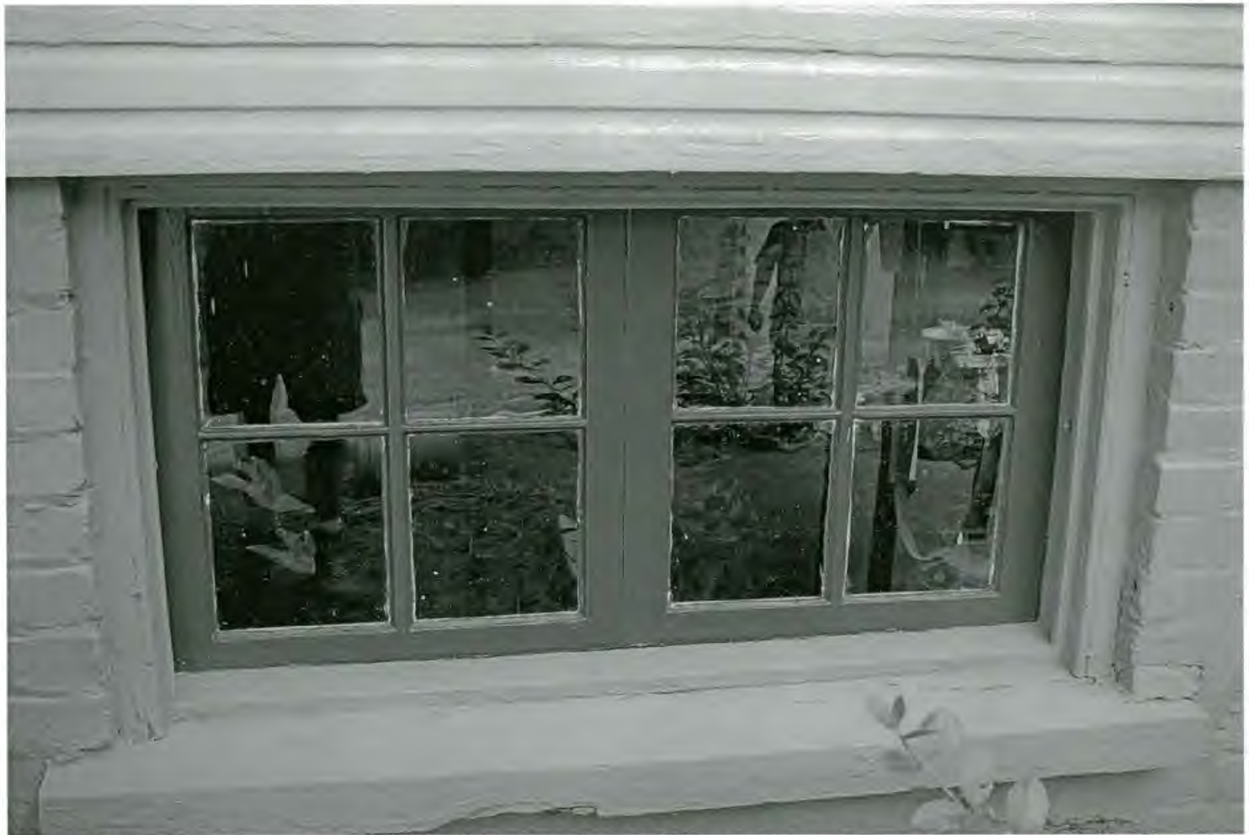
Current view north side bars removed. note 4 lights each, clearly visible from slide 16 8/03/05
