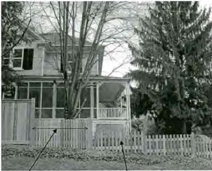
Fence section that should be 3' open picket.style
