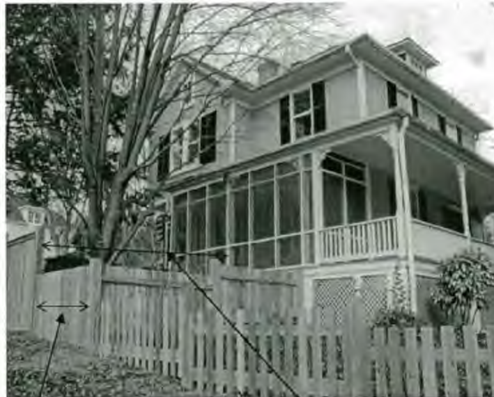
Fence section that should be 3' open picket style
