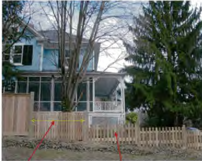
Fence section that should be 3' open picket style
