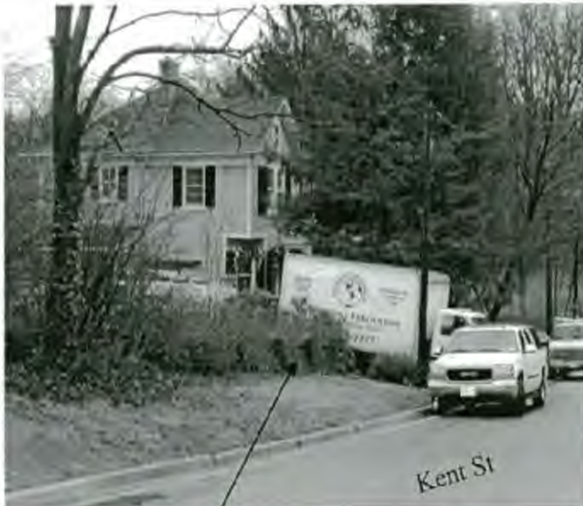
Existing low fence
