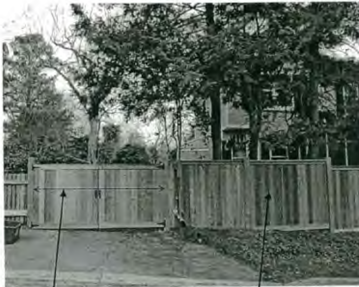
Driveway gate matches privacy fencing rather than tight picket style and is taller than 4'.
