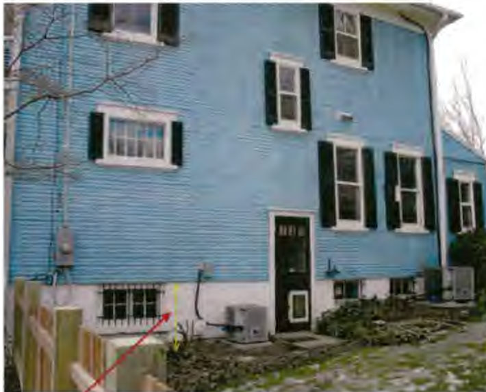
Approximate approved location of Lot 15 side-yard fence
