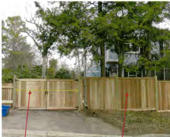
Driveway gate matches privacy fencing rather than tight picket style and is taller than 4'.
