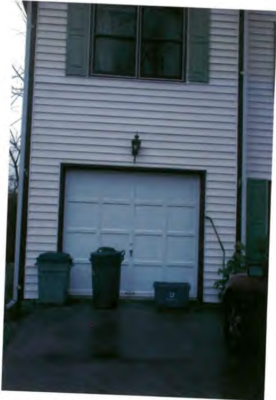
Garage door to be replaced with window
