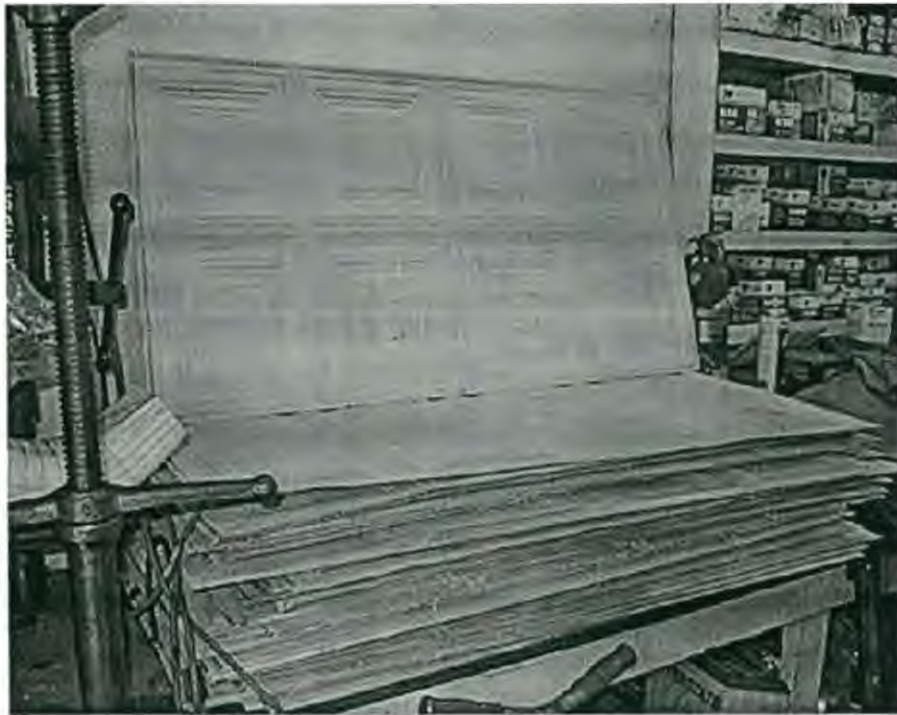
Pressed Metal ceiling panels for 3794 Howard Ave., Kensington Historic District
