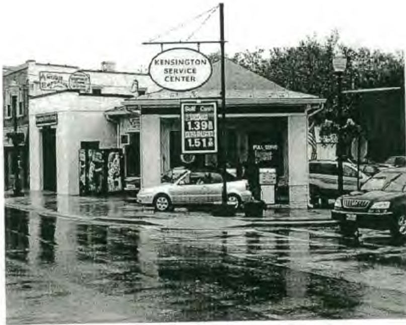
Front elevation of 3794 Howard Avenue
