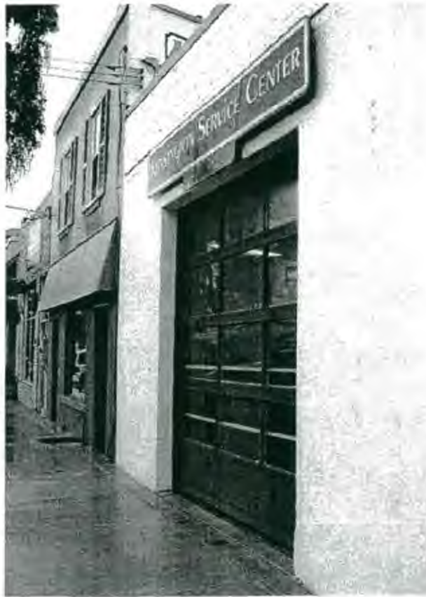
Existing wood roll-up garage door
