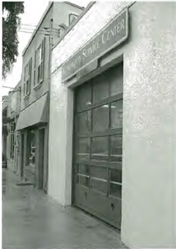
Existing wood roll-up garage door
