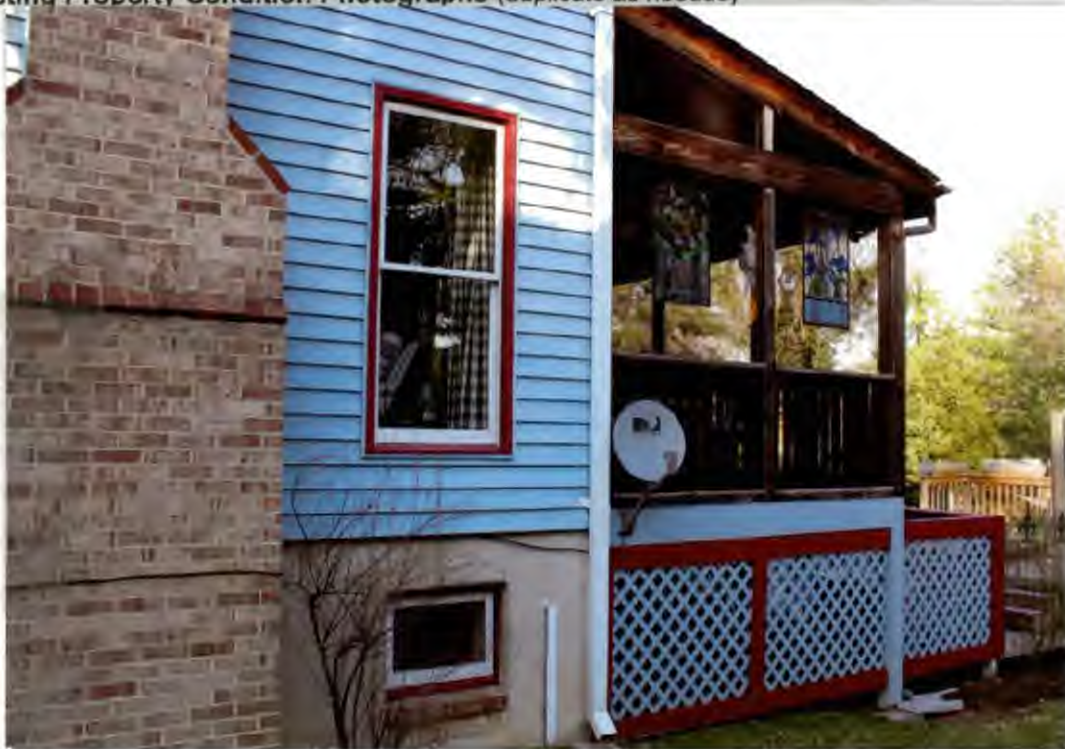
Detail: South facing including porch and deck
