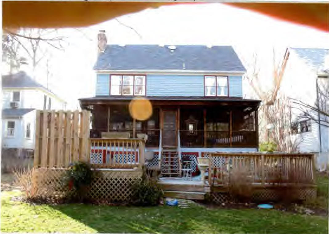
Detail: Looking west (Eastfacing windows)
