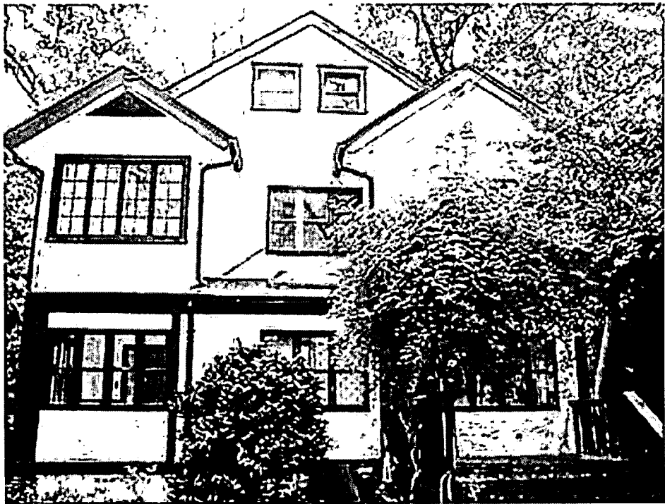
Rear view of property (Note: Boxwood to be relocated in center)
