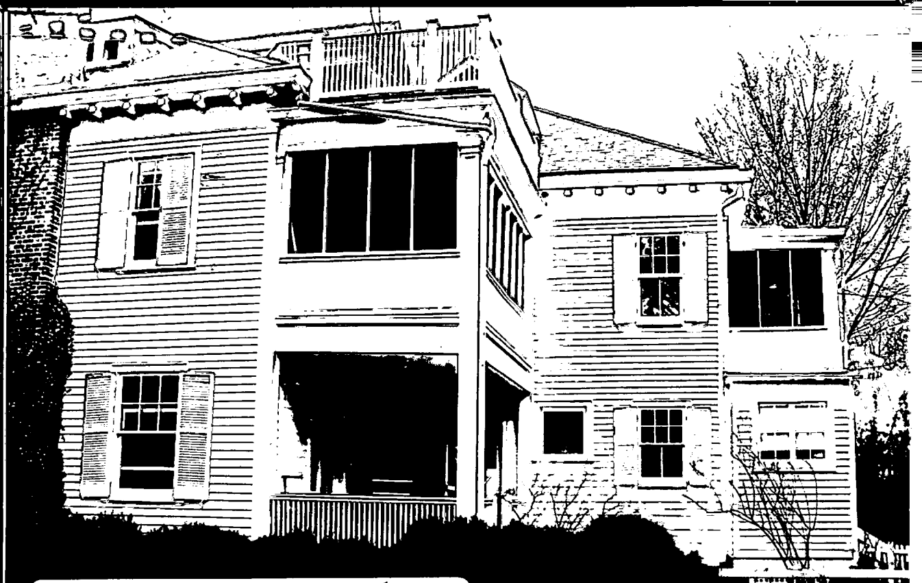
- 10 EAST KIRKE STREET - WEST FACADE, Showing kitchen windows to be removed
