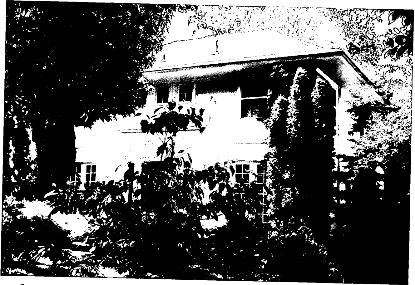
FRONT & RIGHT SIDE, 24 WEST IRVING ST,
