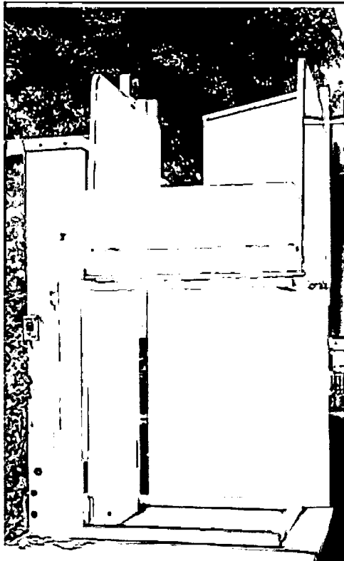
While the lift is in motion, the ramp folds. Once it arrives at a lower landing, one side will lower, allowing easy access.
