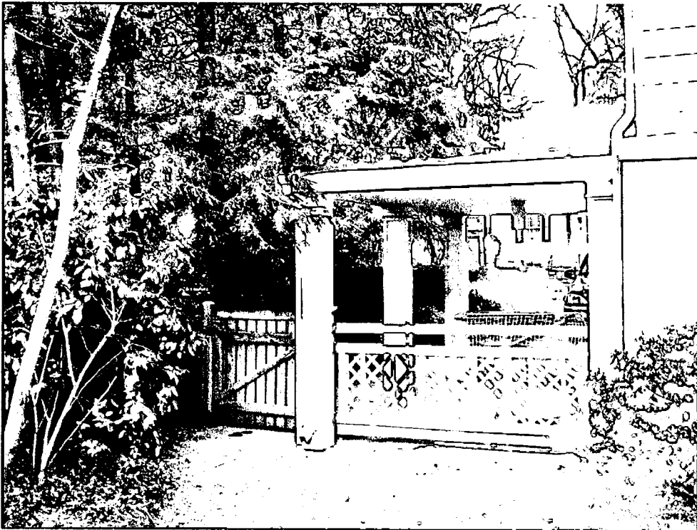
Rear yard fence and gate at carport
