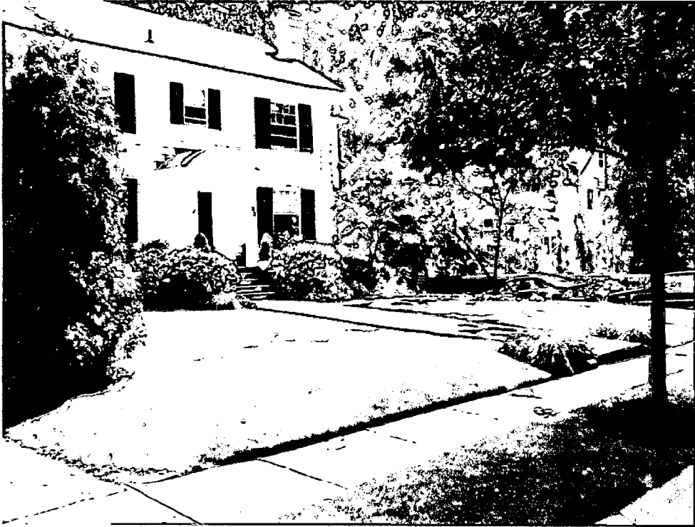
Front Façade approach from the east
