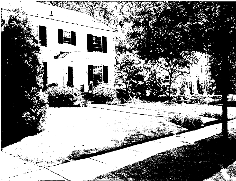
Front Façade approach from the east
