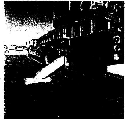
Grasspave 2 's high compressive strength, 5721 psi, make it perfect for green firelanes. A firetruck outrigger will exert only about one-fifth of capacity. Visit our project profiles (put "fire lane" in application field) and view over 70 applications.
