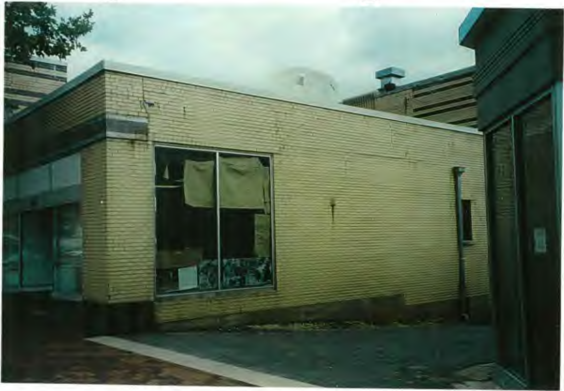
South elevation , west portion.
