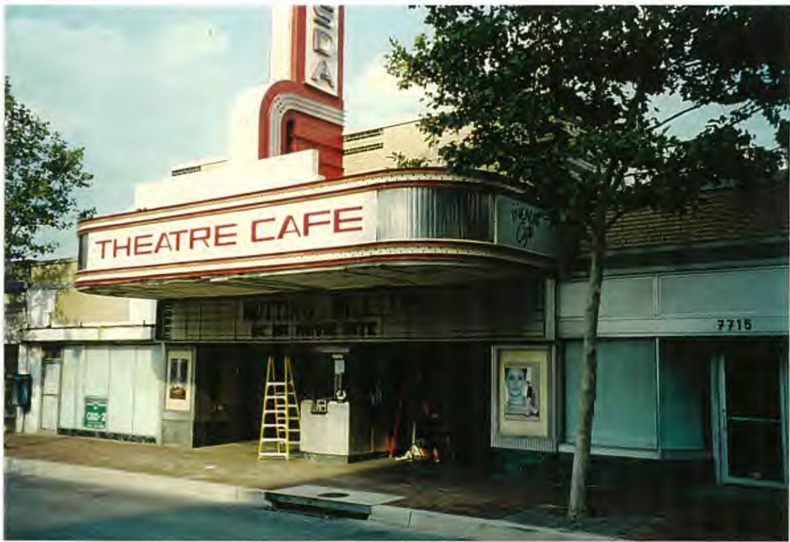
Wisconsin Ave (west) marquee, ticket booth + storefront.
