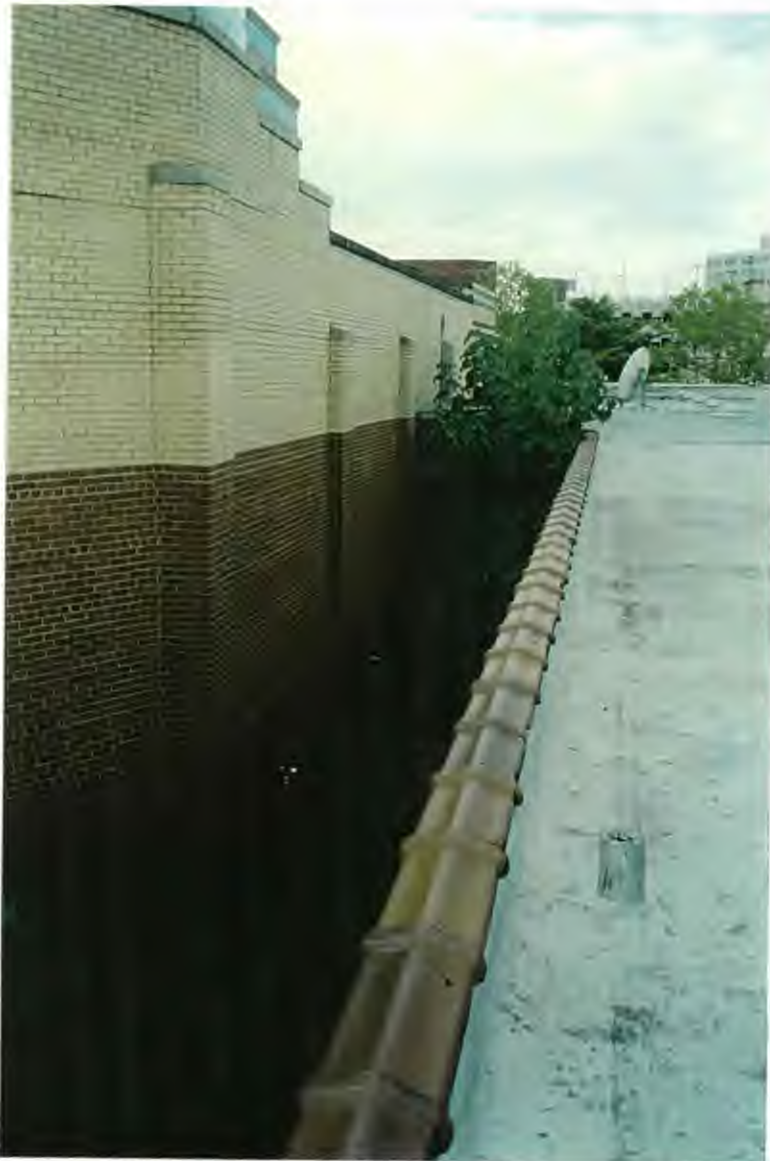
North elevation looking west.
