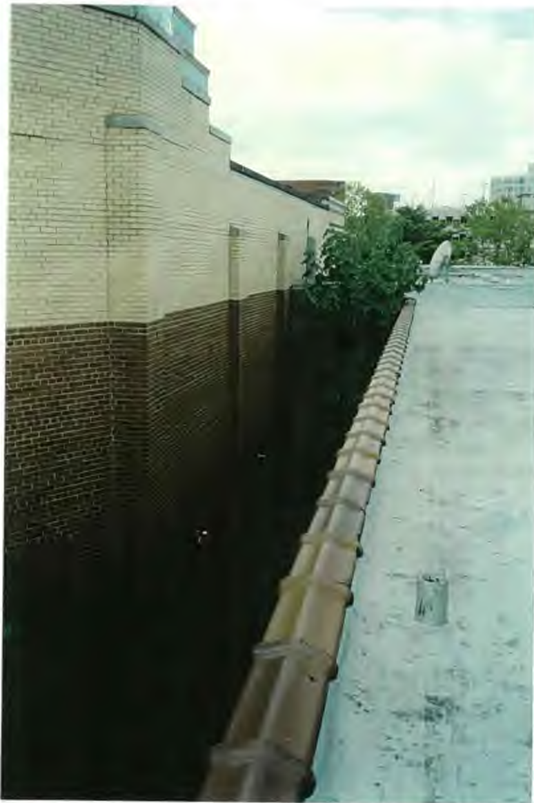
North elevation looking west.
