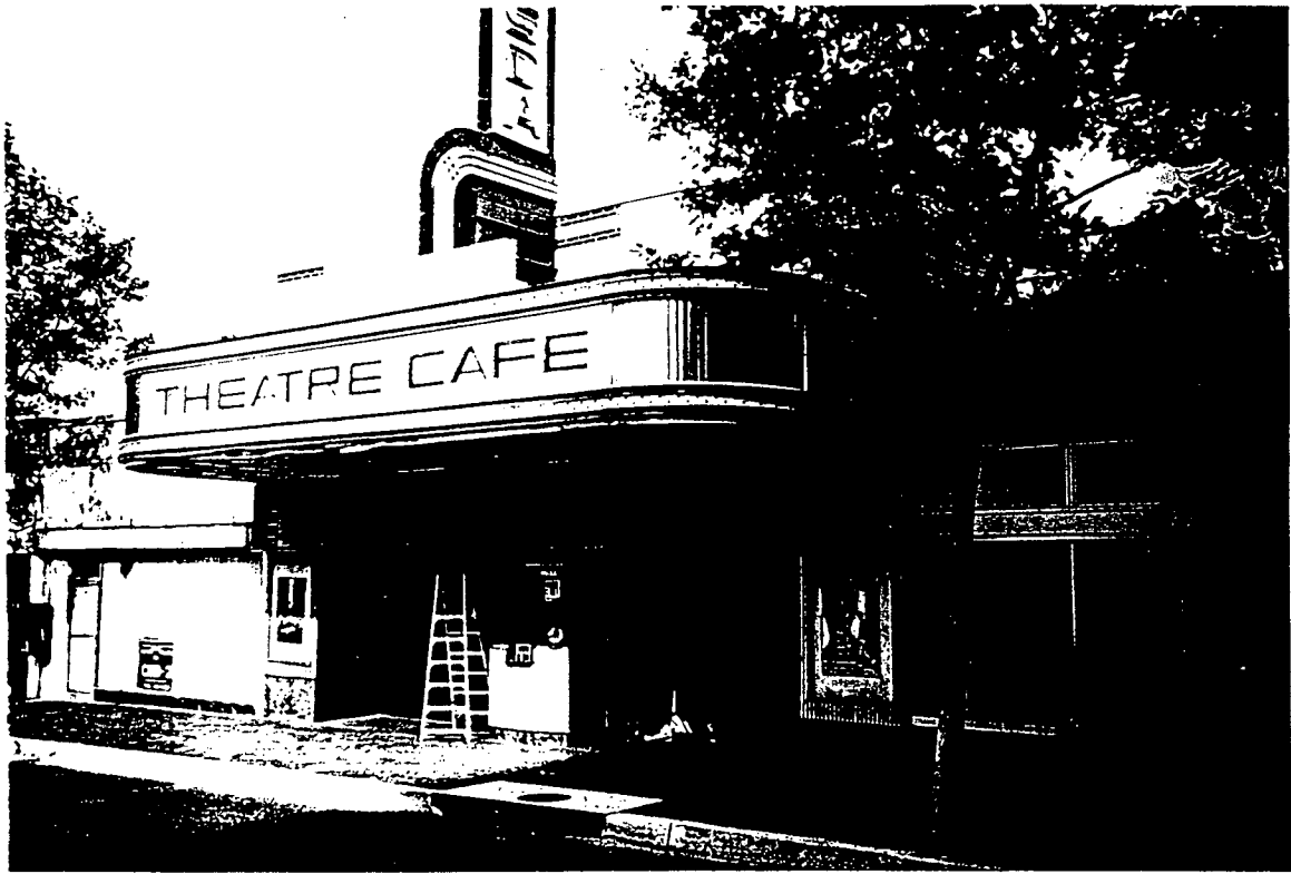
Wisconsin Ave (west) marquee, ticket booth + storefront.
