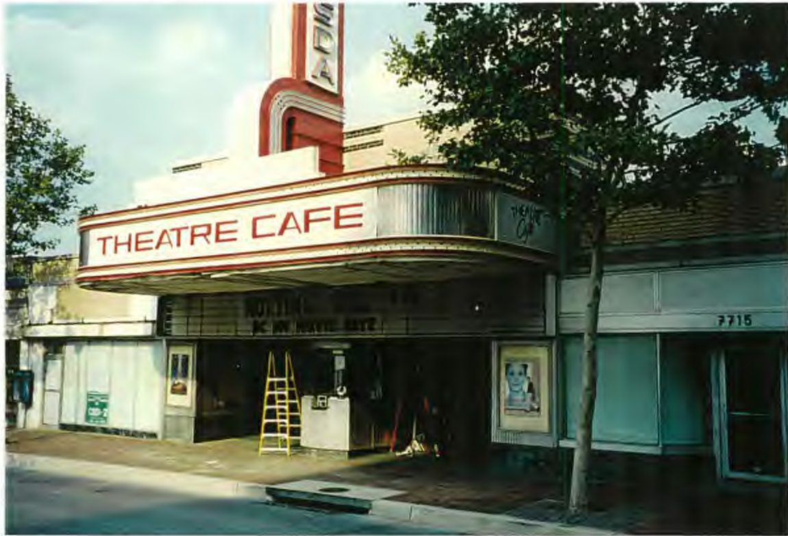
Wisconsin Ave (west) marquee, ticket booth + storefront.
