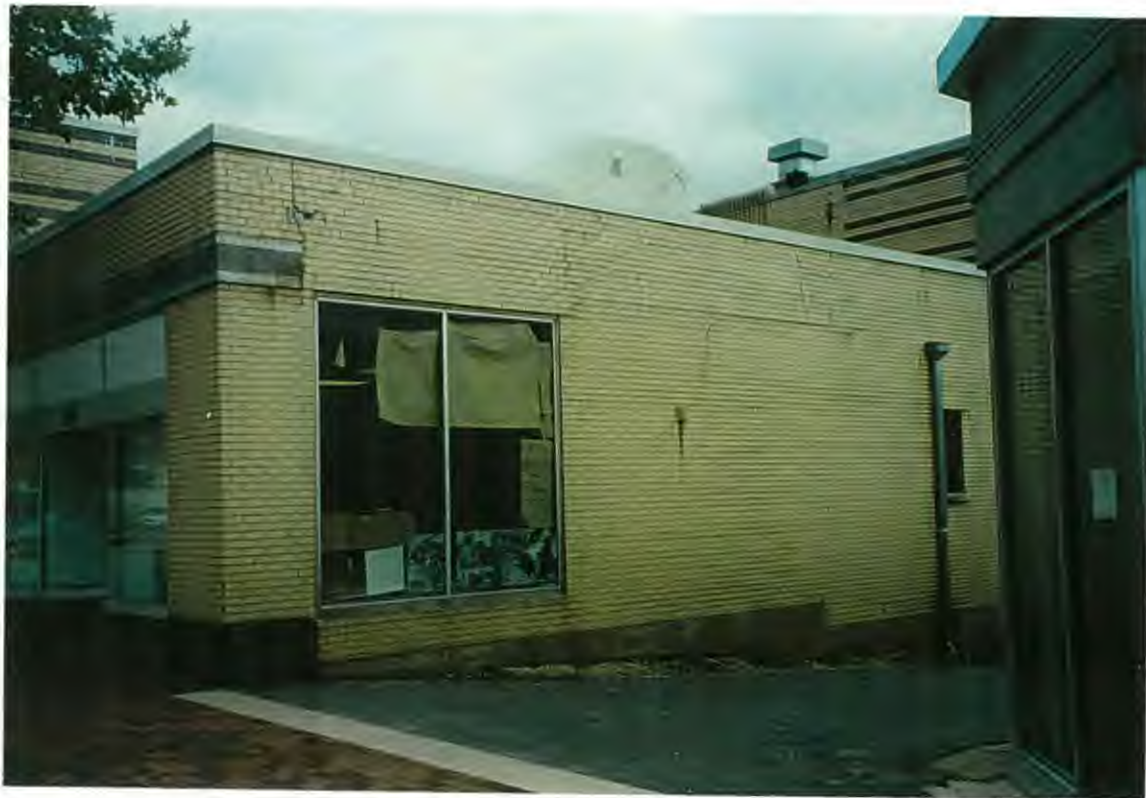
South elevation, west portion.
