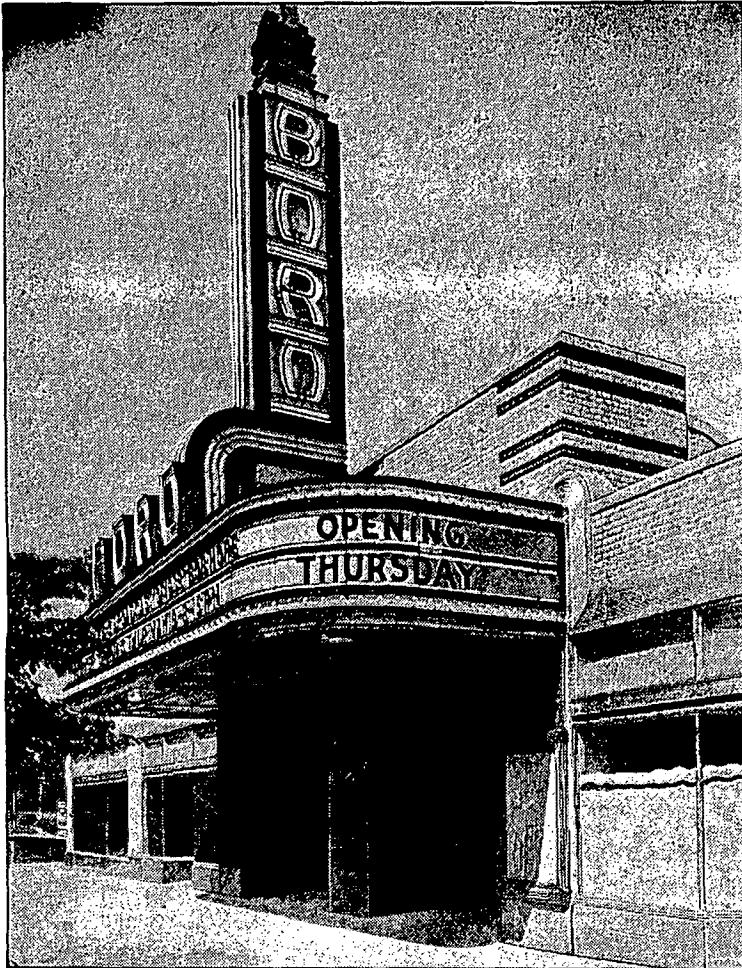
Boro Theatre, the last word in theatre construction, which will be opened here Thursday night with an impressive program beginning at 8:15 o'clock. The new amusement palace boasts the latest in sound and projection equipment and is fitted with ultra-modern features for the comfort of its patrons. The theatre will operate under the direction of Sidney Lust, head of a large chain of theatres in Washington, Maryland and Virginia.
