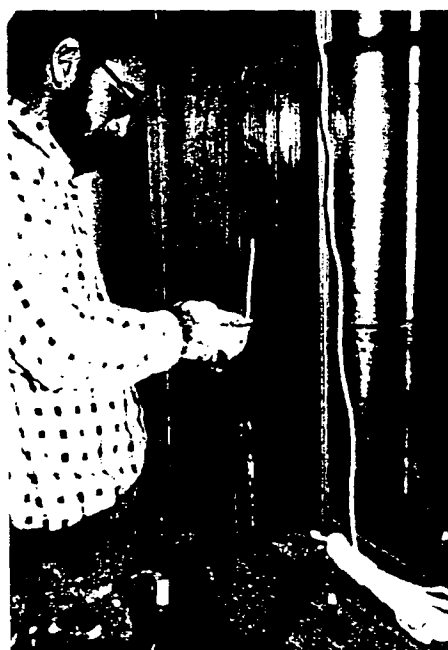
Figure 4e. A common repair is the replacement of broken sash cords with new cords (shown) or with chains. The weight pocket is often accessible through a removable plate in the jamb, or by removing the interior trim. Photo: John H. Myers
