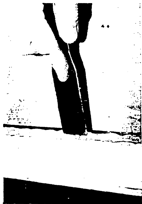
Figure 4d. Reglazing or replacement of the putty requires that the existing putty be removed manually, the glazing points be extracted, the glass removed, and the back putty scraped out. To reglaze, a bed of putty is laid around the perimeter of the rabbet, the pane is pressed into place, glazing points are inserted to hold the pane in place, and a final seal of putty is beveled around the edge of the glass. Photo: John H. Myers
