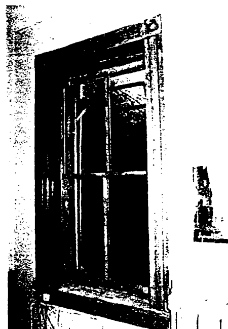
Figure 4f. Following the relatively simple repairs, the window is weathertight, like new in appearance, and serviceable for many years to come. Both the historic material and the detailing and craftsmanship of this original window have been preserved. Photo: John H. Myers
