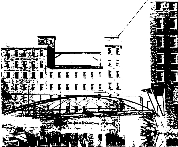
Figure 1. Windows are frequently important visual focal points, especially on simple facades such as this mill building. Replacement of the multiple windows here with larger panes could dramatically change the appearance of the building. The areas of missing windows convey the impression of such a change. Photo: John T. Lowe
