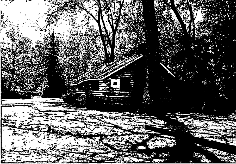
Cabin from north side showing concrete pad to be removed.
