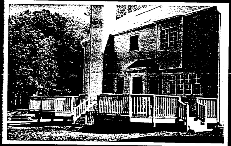
DECK—with railing and steps
